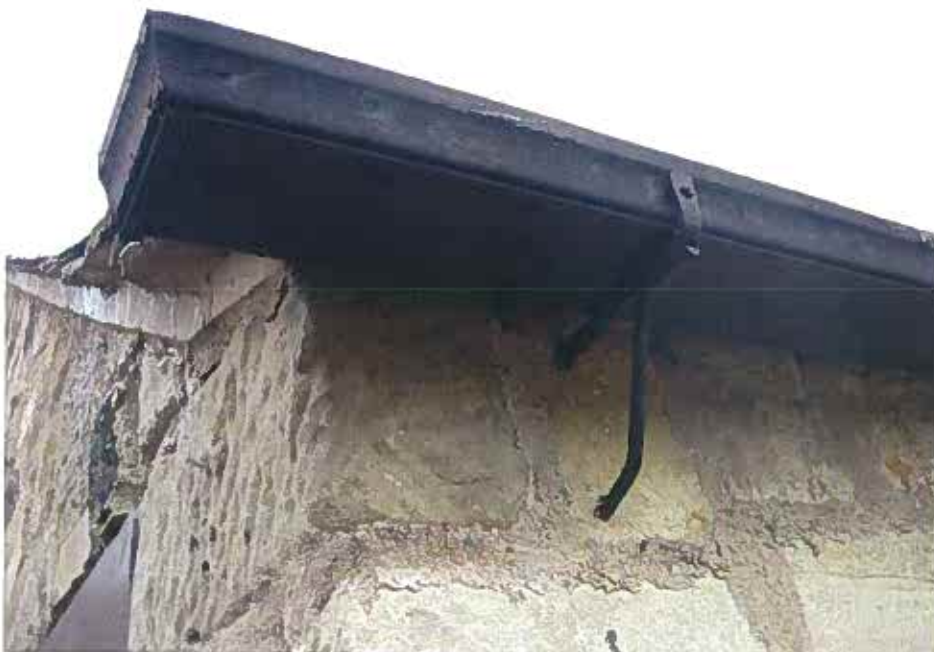
Wooden Guttering and Metal Brackets Shown On Garage
