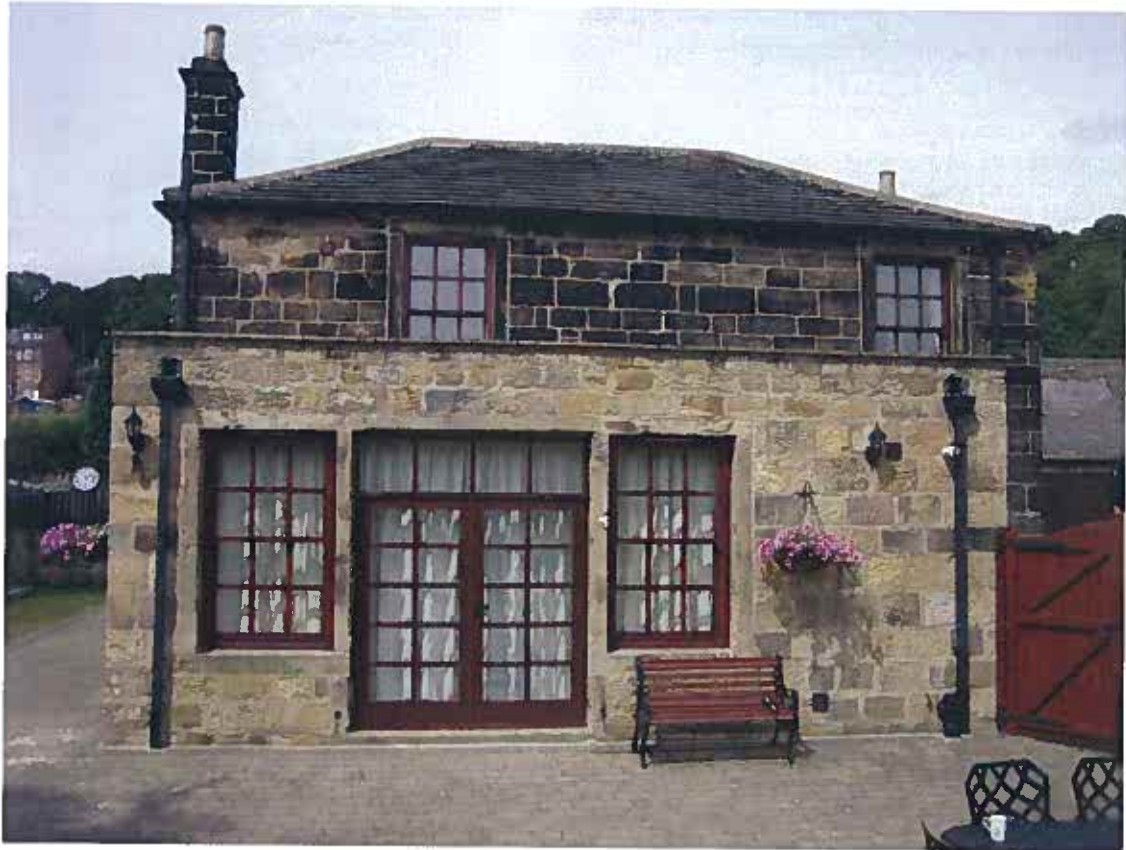
Modern Extension With Flat Roof and Parapet as Proposed Solar Panel Location
