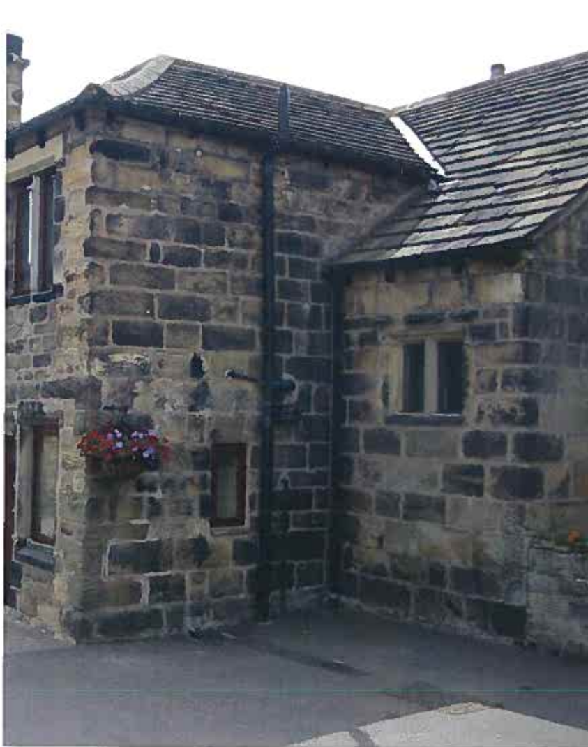
Windows in question shown to right of picture under Cat Slide roof
