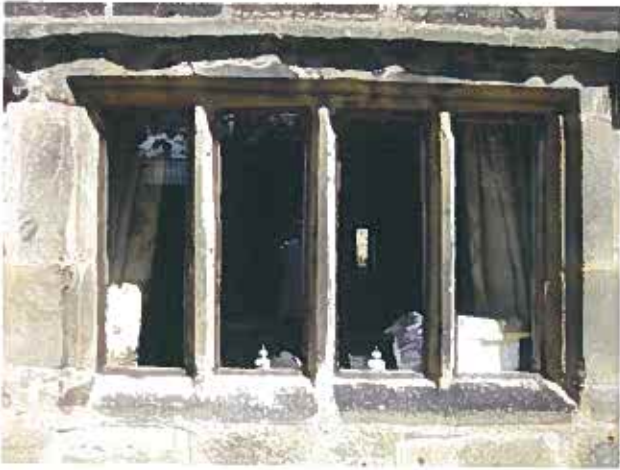
Existing Dining Room Windows
