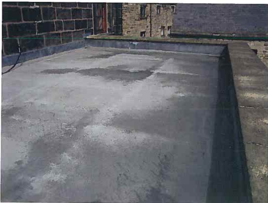
Photo Showing Flat Roof and Extent of Parapet
