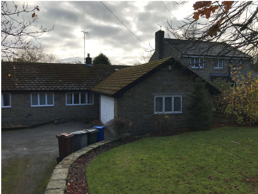
Fig 02. Front north elevation and garage
