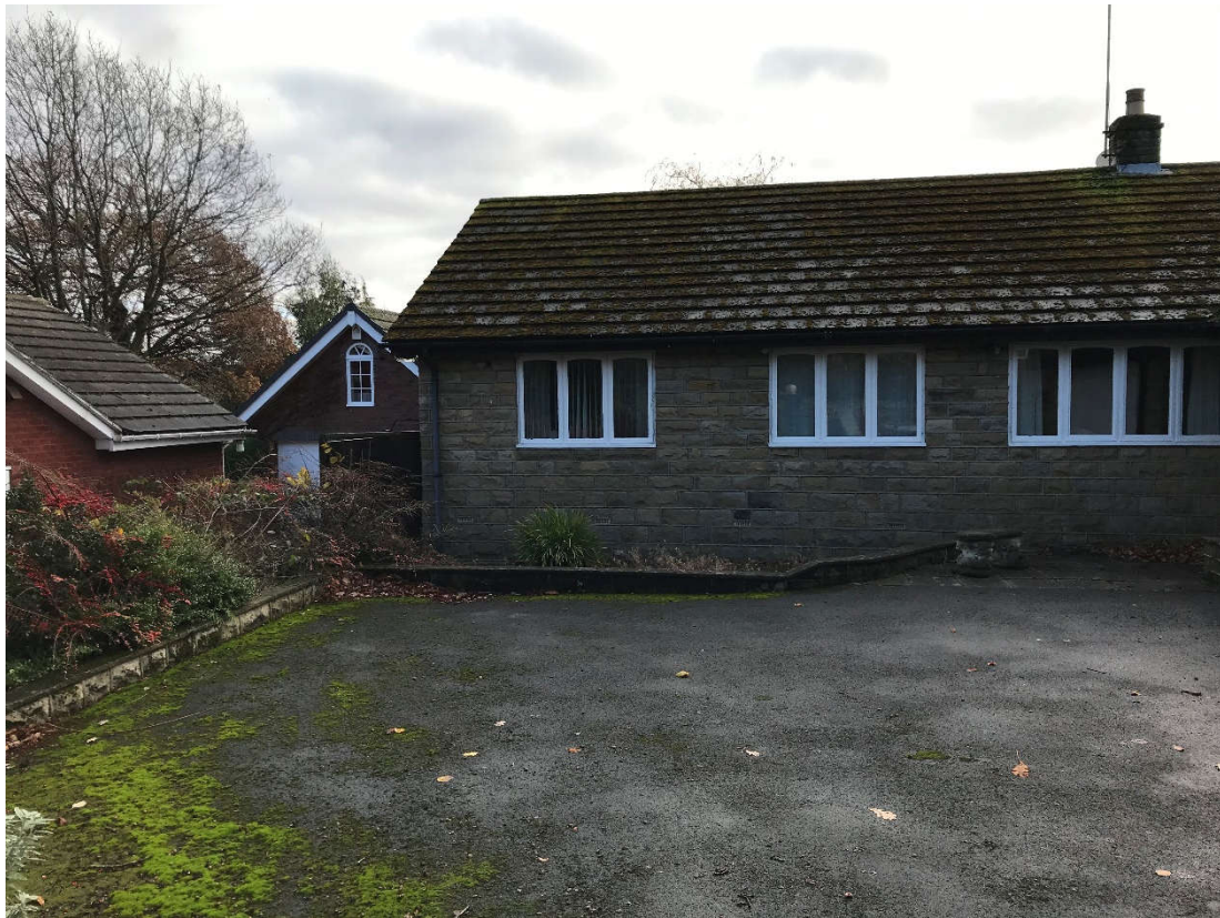
Fig 01. Front north elevation
