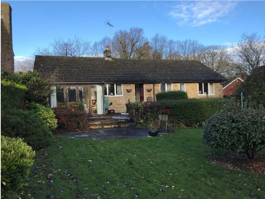
Fig 03. Rear south elevation and terrace.
