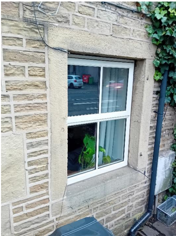
Figure 4. 8 Thurlstone Road Front Ground Floor window
