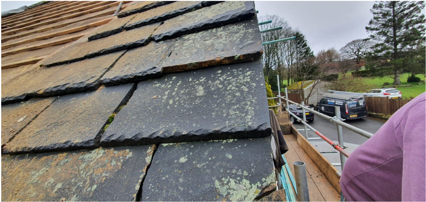
Reclaimed stone roof tiles
