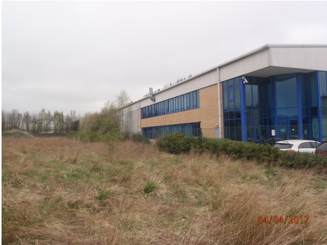
Photo 5 - North-easterly view of the hedgerow and fenced perimeter of the site. Pilkington AG is present directly east of the site.
