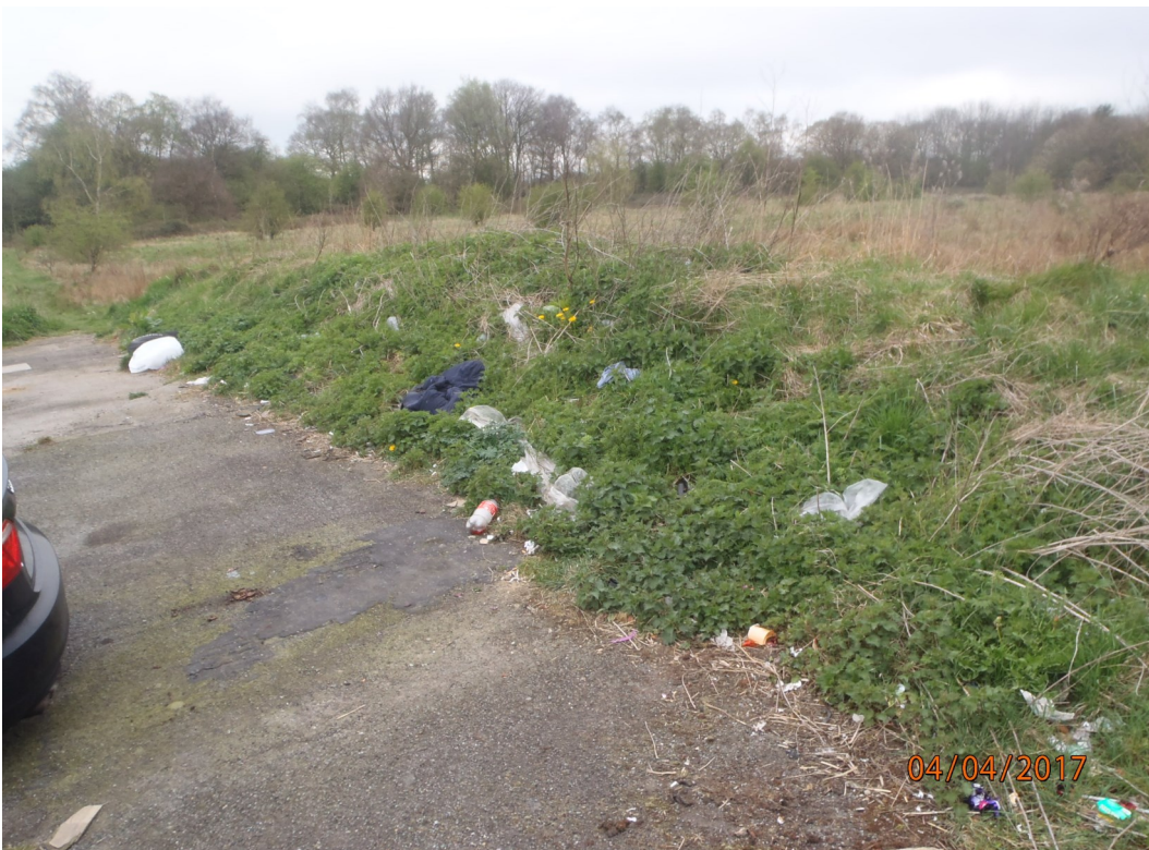
Photo 2 - North-westerly view of the bund at the southern boundary of the site and the site entrance in the corner of the image. Litter is prominent in this area.
