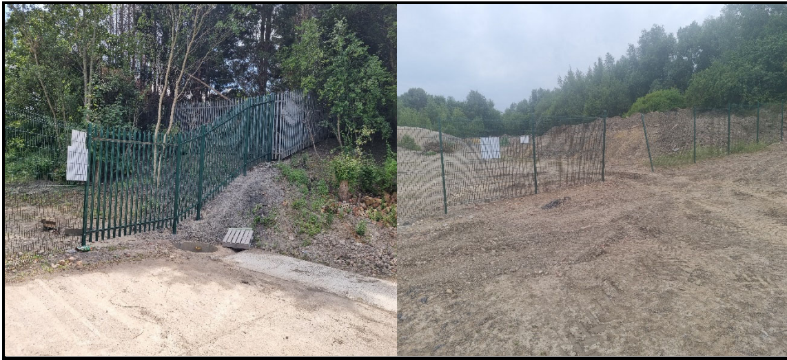
Completed fencing along southern and northern site boundaries.
