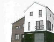
3 Storey & 2 Storey Combination House
