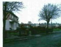
Feature 1 - Domestic Property
