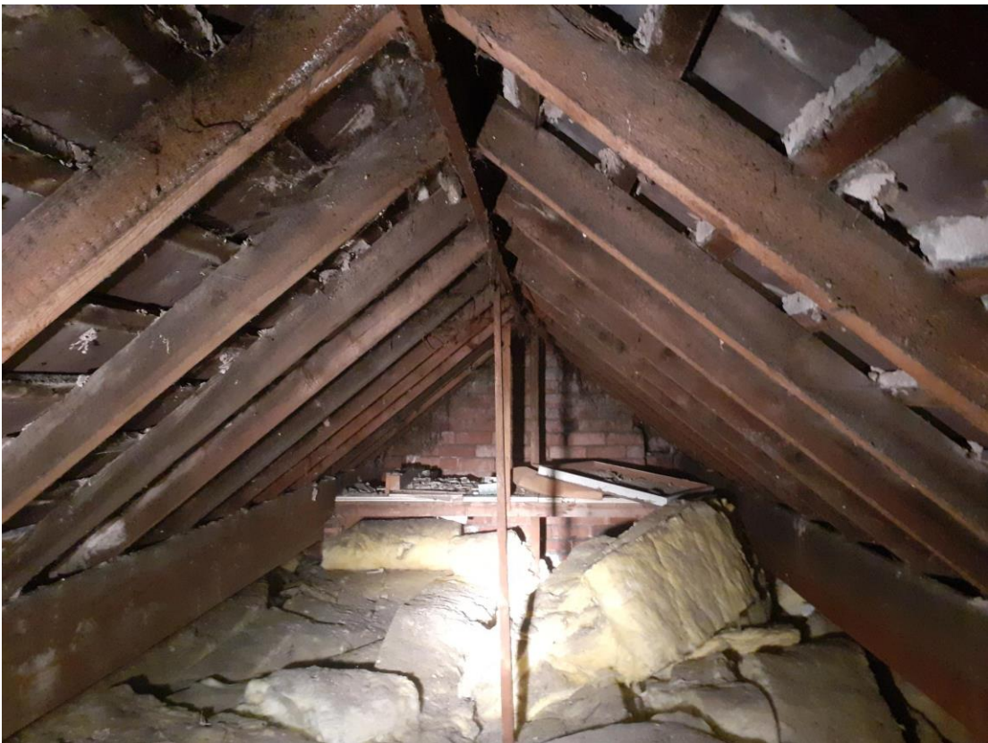
Plate 5: Underside of roof tiles (no membrane or sarking) of the gable end extending outwards to the 'left' (south) of the single-storey extension pictured in Plate 3.
