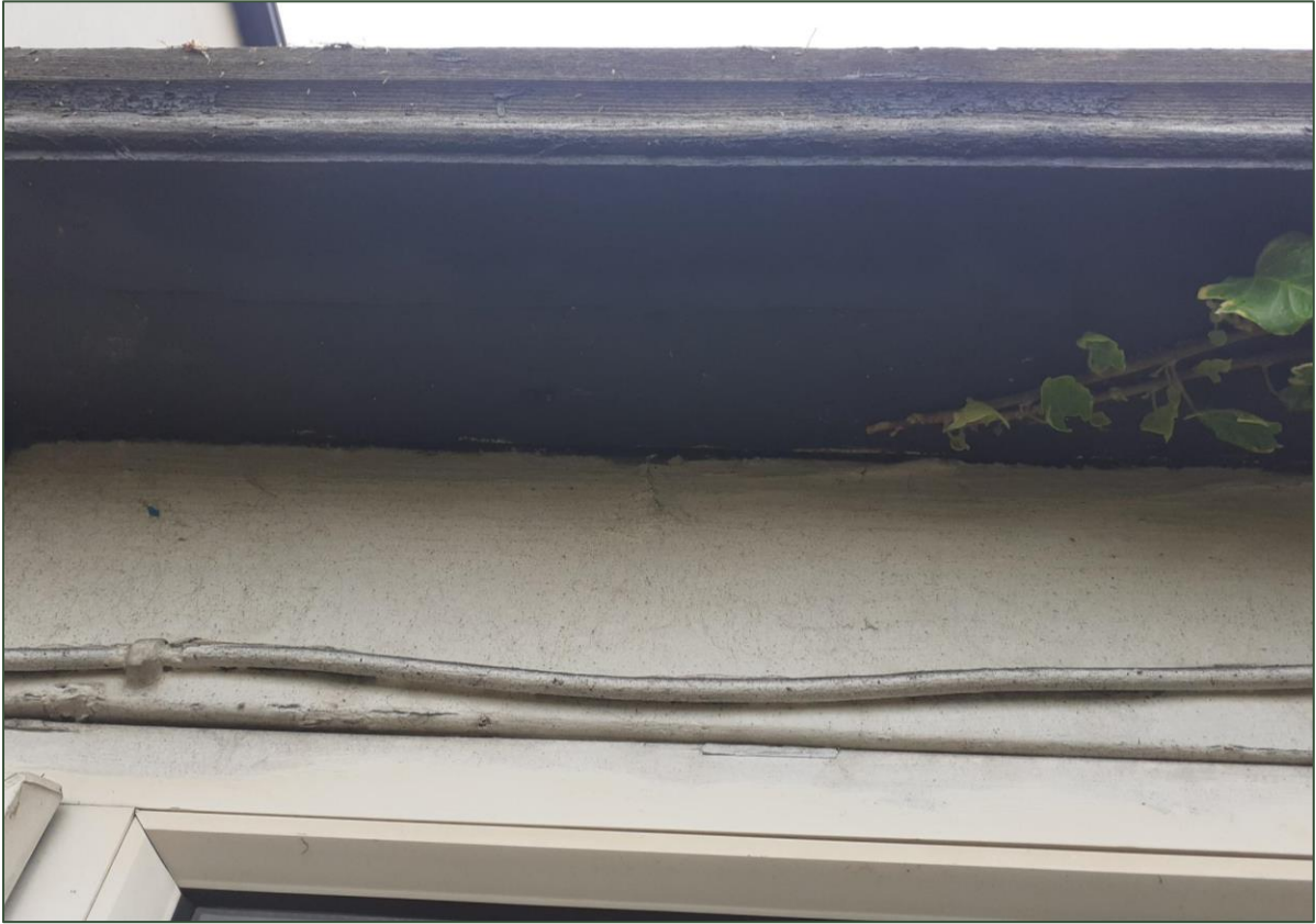
Plate 2: Tightly-fitting wall of single storey extension, at eaves level.
