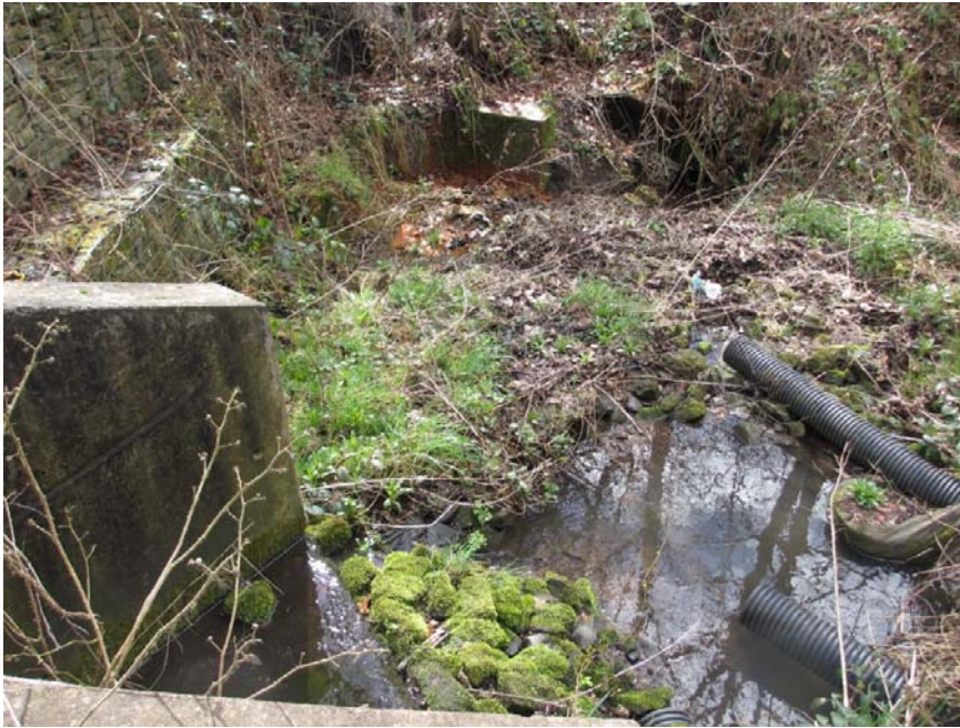
Northern Site – Culverts coming together north west of site
