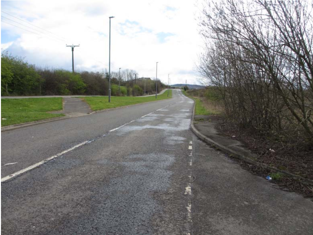
Northern Site – View looking south from existing access shown low spot in road
