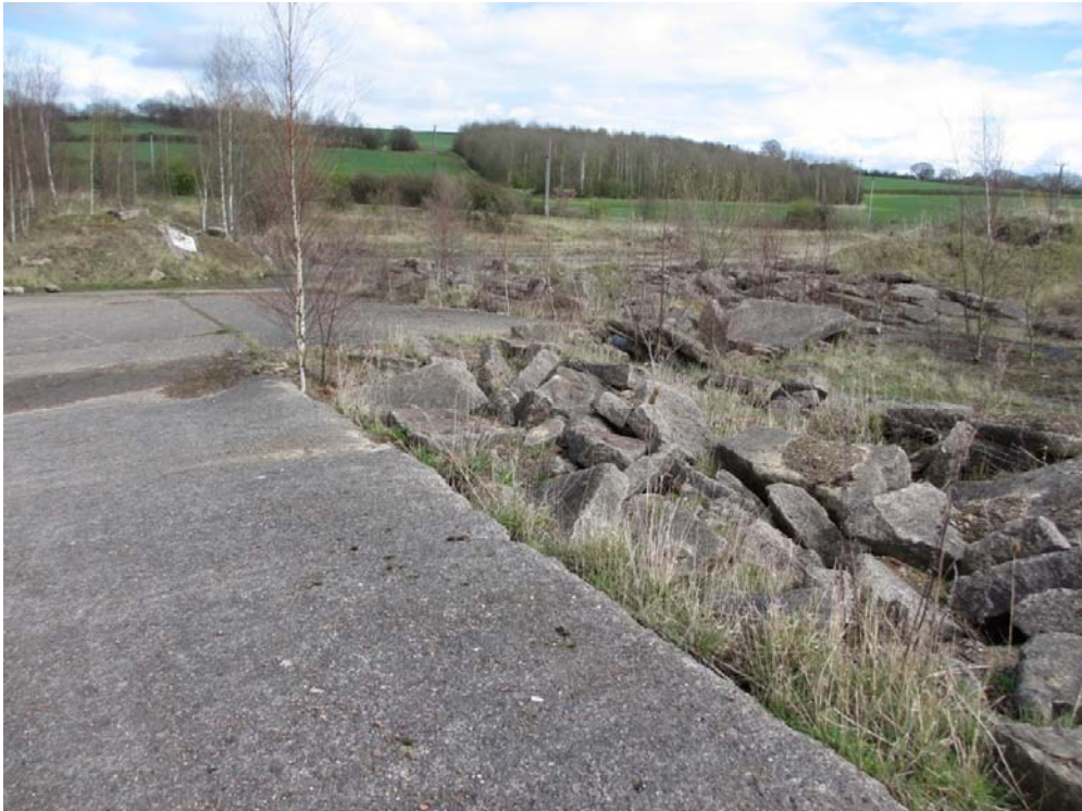
Northern Site – Centre of site looking East towards Woolley Colliery Road
