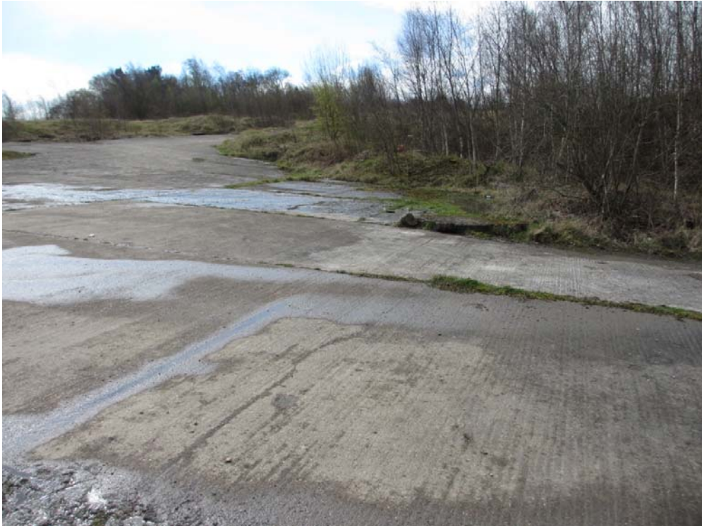
Northern Site – View across centre of the site showing hardstandings
