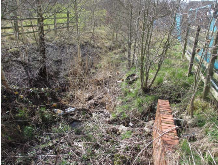
Northern Site - Open Watercourse to northern boundary
