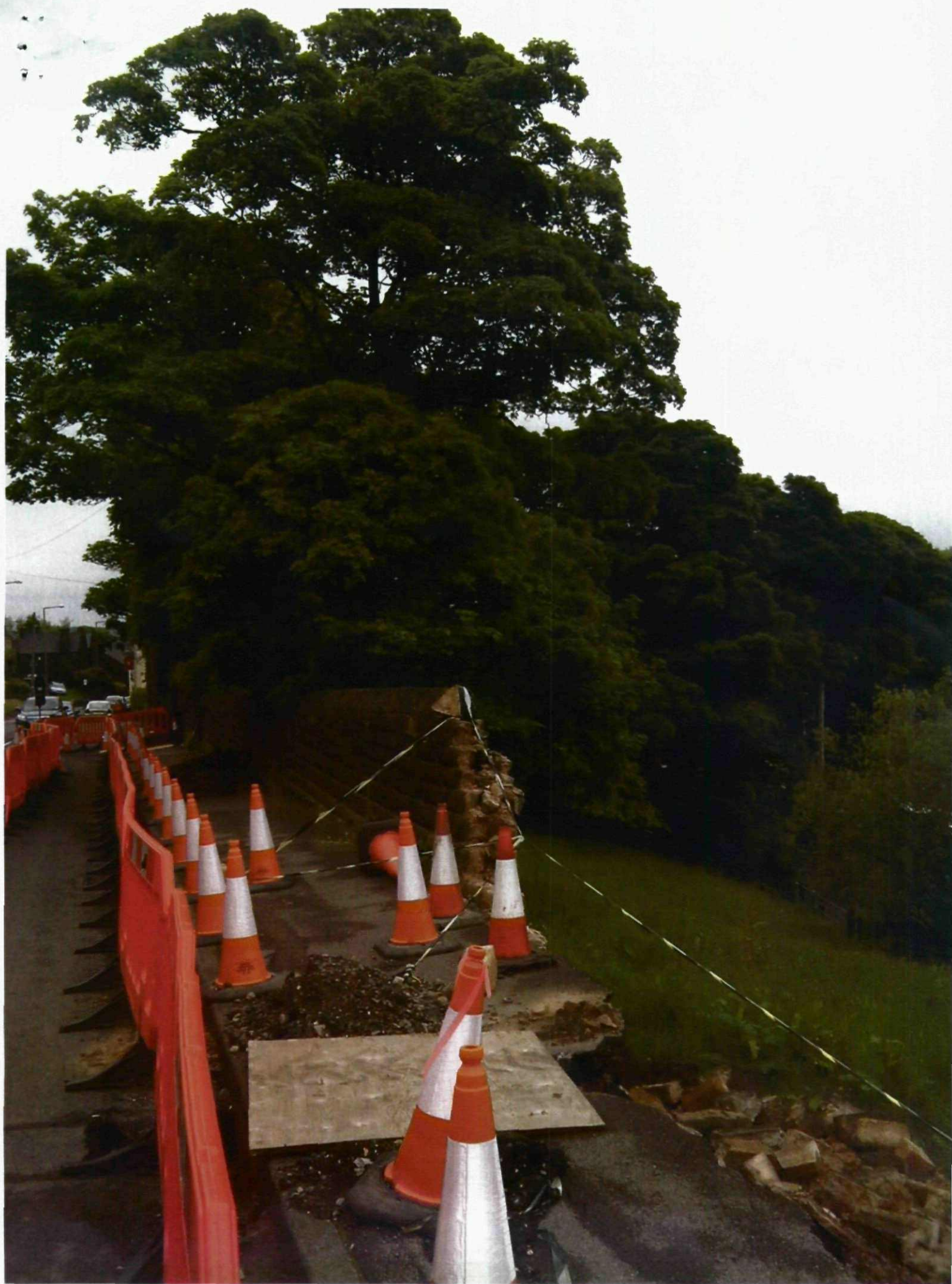
MANCHESTER ROAD; TUNNEL ZONE.
