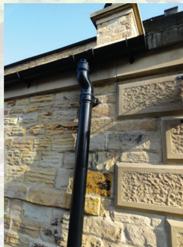
Wrought Iron rain water gutters and downpipes. Rusticated quoins.
