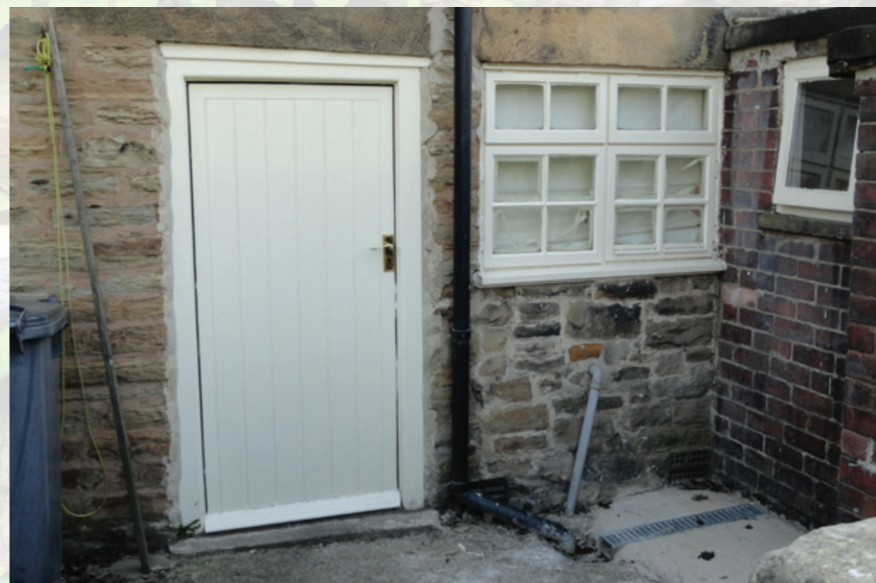
Traditional timber frame door and window in Elsecar.
