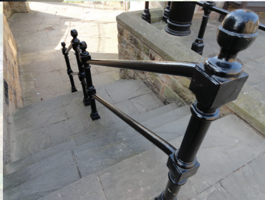
Wrought Iron balustrading and stone steps.
