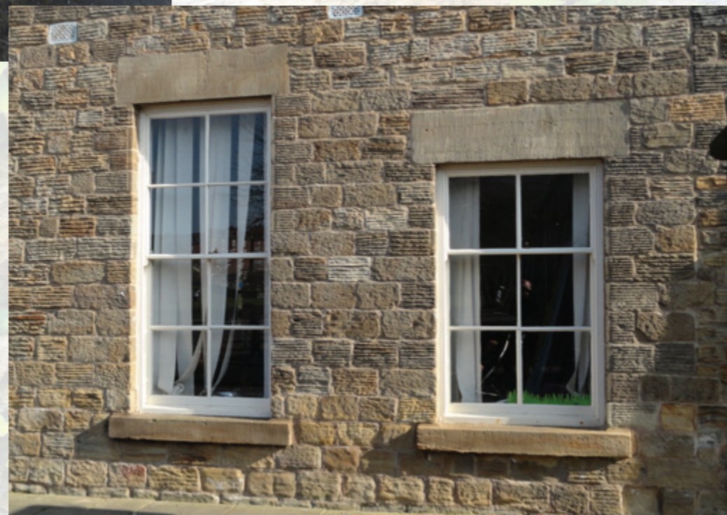
Traditional timber frame windows & stone walling.
