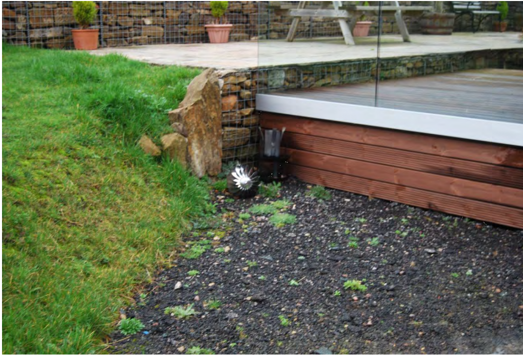
Photograph number 7 showing the excavation depth for the tiered area to the rear of the slab for the house and the paved area construction in support of gabion wall so the excavation is benched and then sealed by the paving to avoid water ingress into the stratum.
