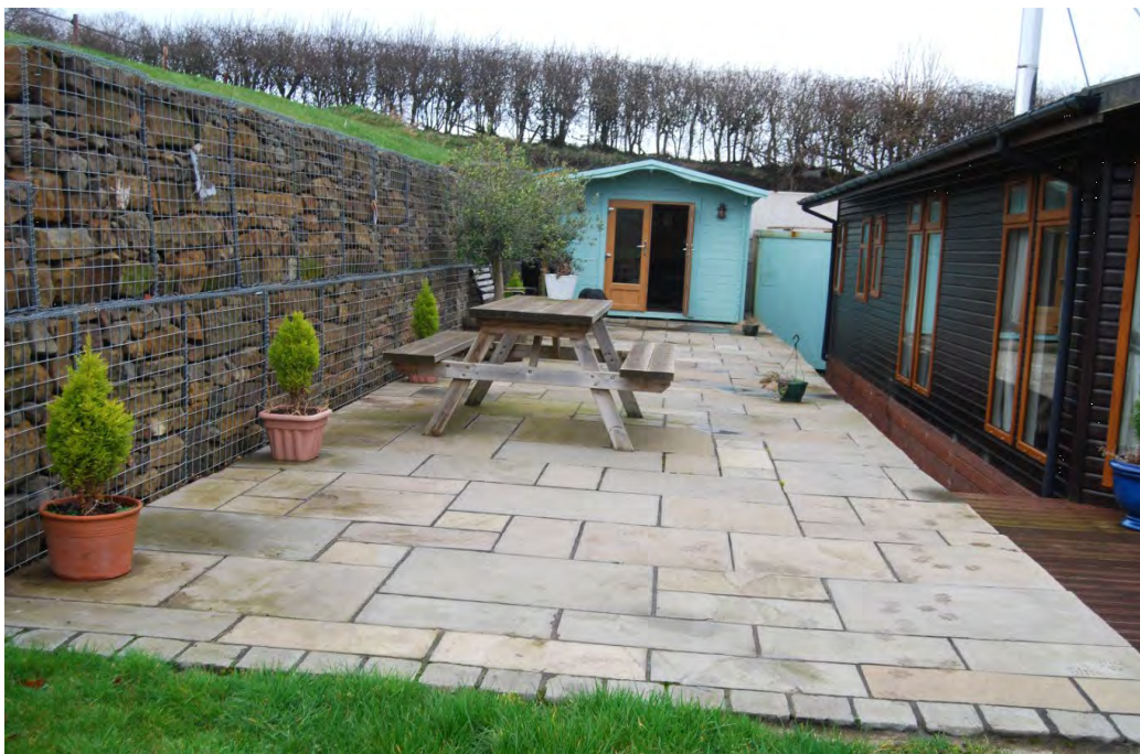
Photograph number 8 showing the upper gabion wall founded on the concrete strip footing and slab then paved to prevent water ingress into the mudstone beneath. The paved area is covering the gabion wall to support the excavation in mudstone for the house and provides a lateral force on the upper gabion wall foundation. The small wooden structure is a tack room and office for the business and is hidden from view in the landscape. The paved area and tack room are used for visiting guests to the livery stable and rare breeds farm.
