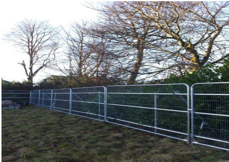
Picture 1. Example of BS5837:2012 Protective Fencing
