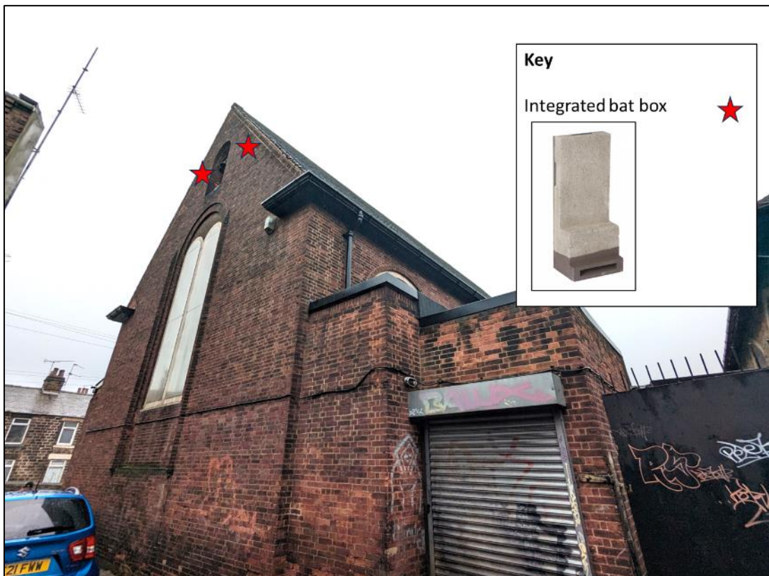
Figure 3. Recommended locations for integrated bat boxes
