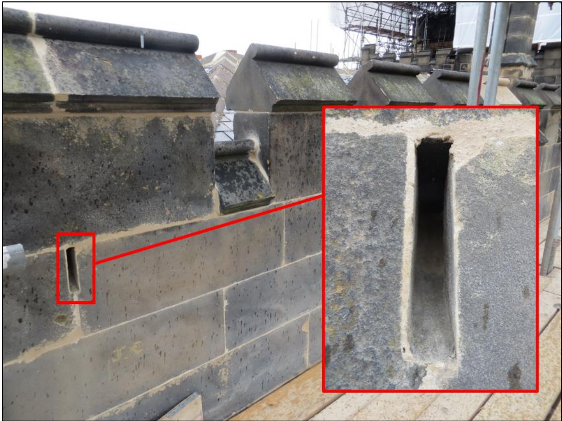
Plate 13. Example of mortar being used to create a ramp at base of a prospective roost location to let water out
