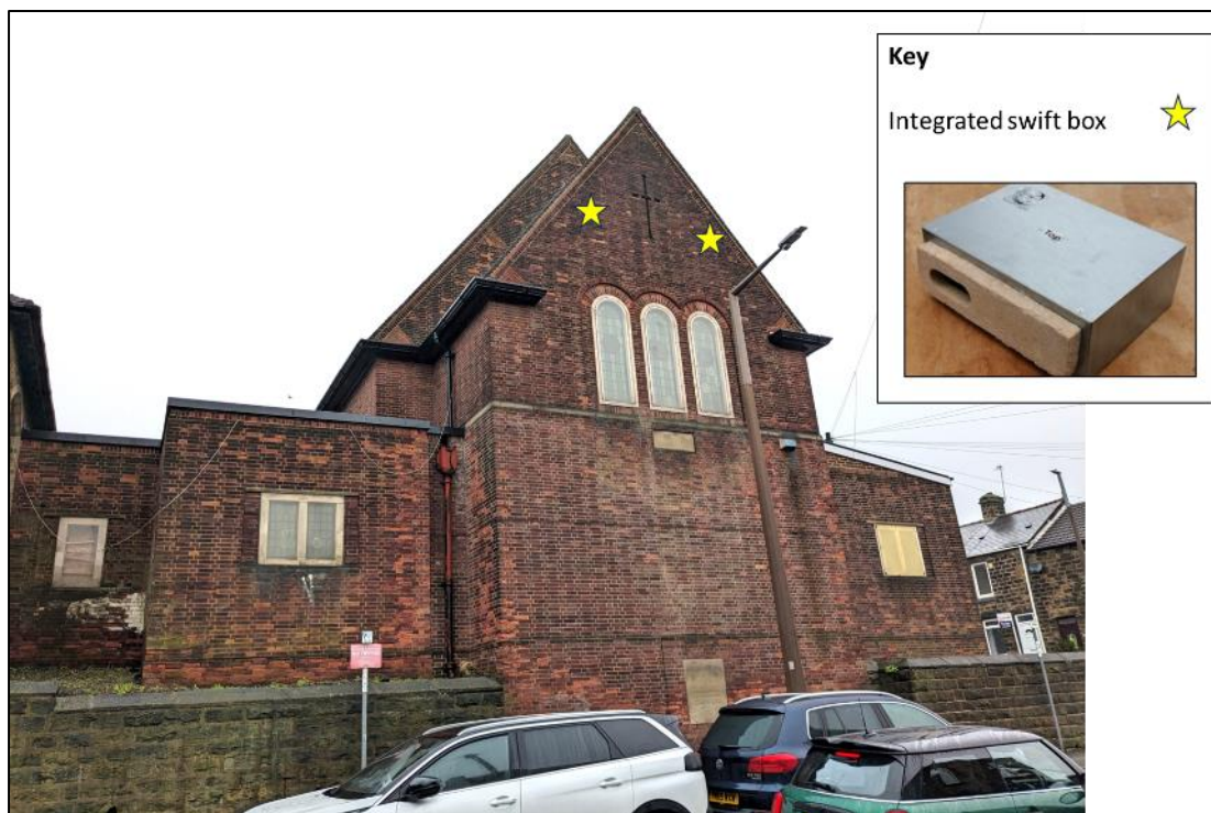
Figure 4. Recommended locations for integrated swift boxes
