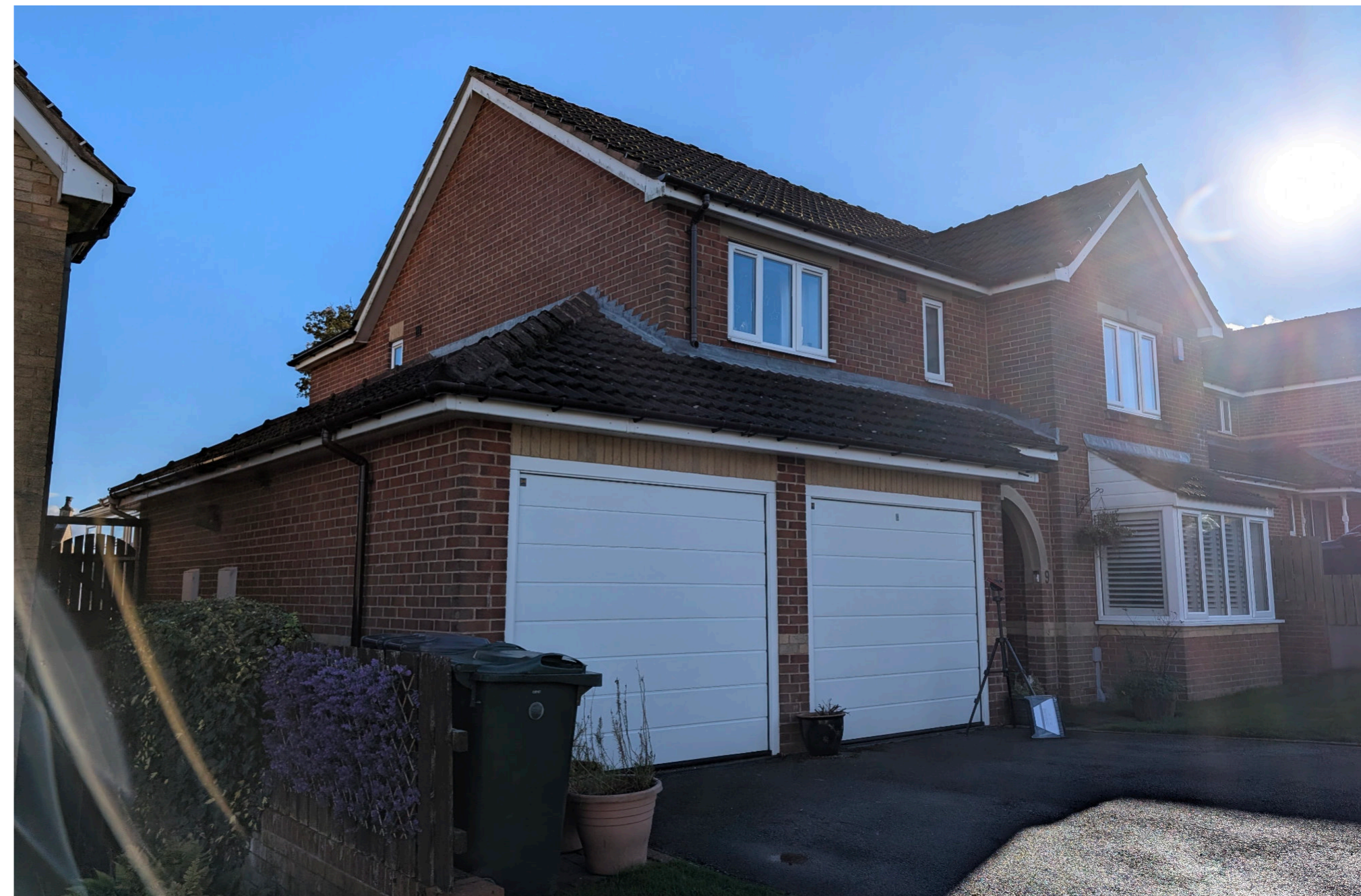
2509 - 9 Kirkhill Bank, Cubley, Penistone, Sheffield, S36 9UX Existing NE (side) Elevation
