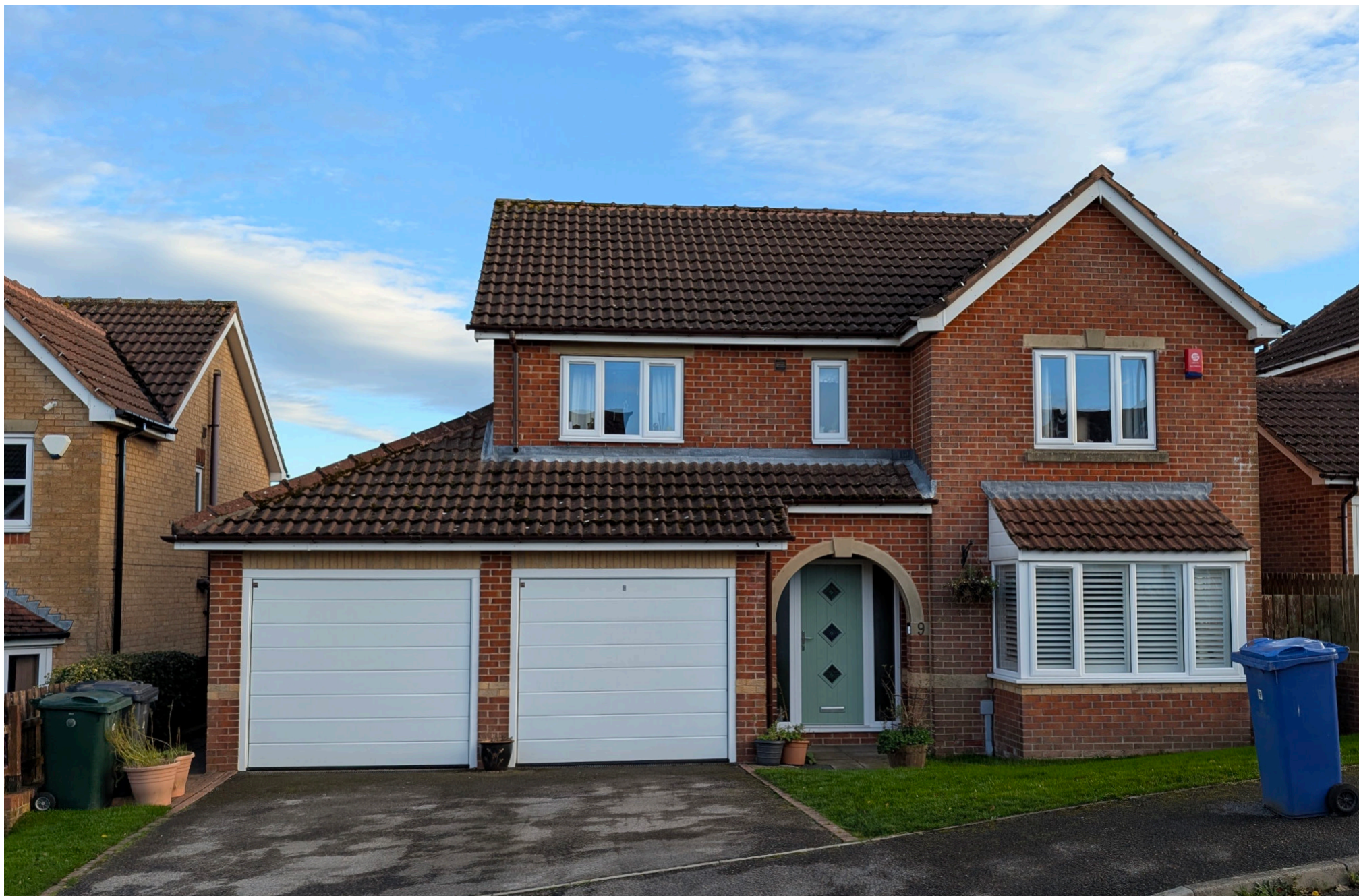
2509 - 9 Kirkhill Bank, Cubley, Penistone, Sheffield, S36 9UX Existing NW (front) Elevation
