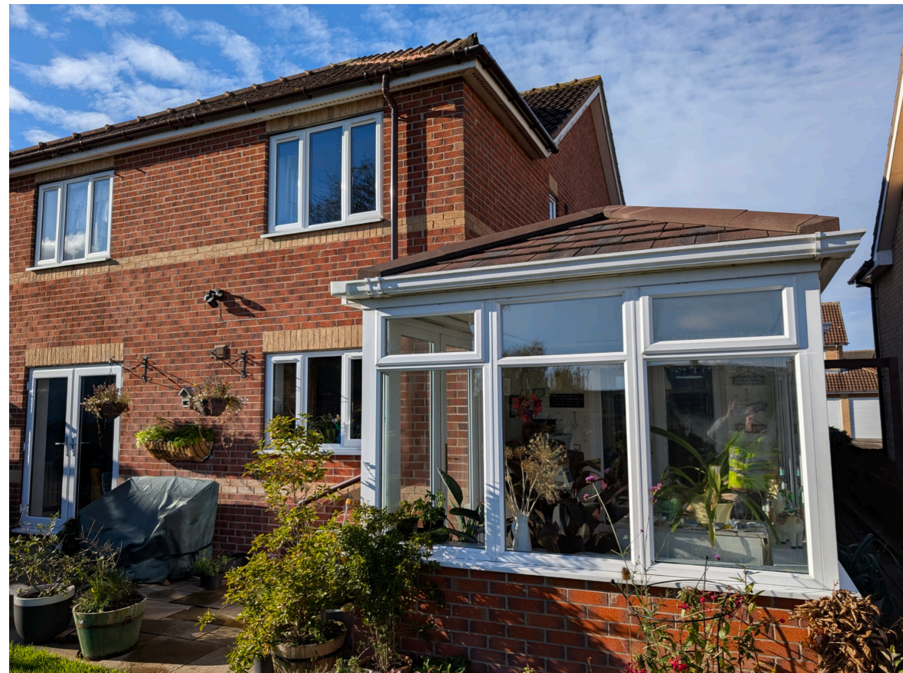
2509 - 9 Kirkhill Bank, Cubley, Penistone, Sheffield, S36 9UX Existing NE (side) Elevation
