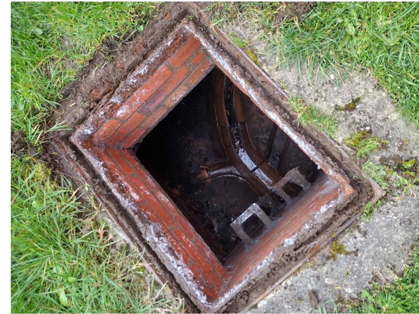
Existing Inspection Chamber 1
