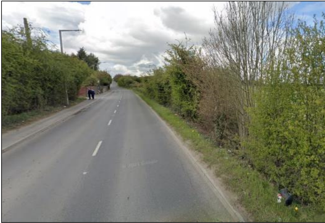
Figure 3-3 Existing Footway on Shaw Lane (Source: GOOGLE)
