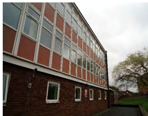
Figure 7. Southern aspect of Building 2 with plastic cladding surrounding windows.
