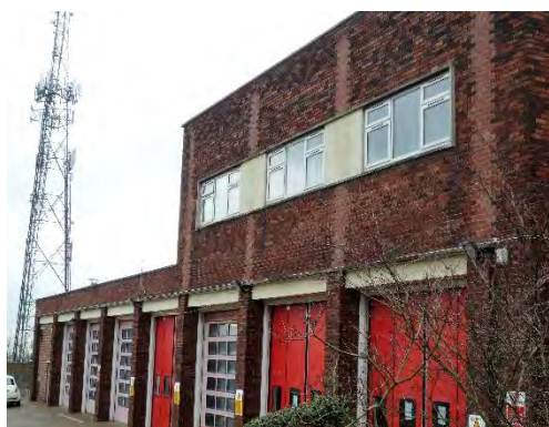
Figure 4. Western aspect of Building 1 with fire engine garages.
