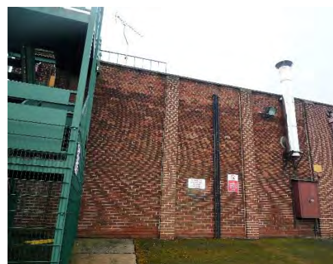
Figure 5. Eastern aspect of Building 1 with intact brick walls and flat roof.
