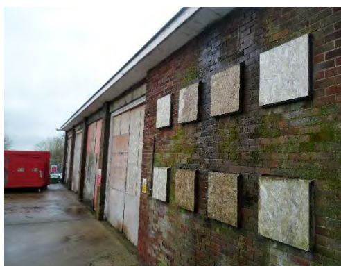
Figure 10. Western aspect of Building 4 with bricked up windows and garage doors, showing wooden soffit box and flat bitumen roof.
