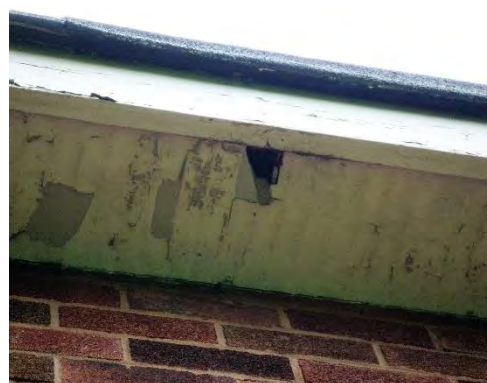
Figure 9. PRF on southern aspect of Building 3 within soffit box.
