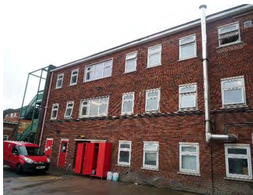
Figure 6. Northern aspect of Building 2 including fire service offices.
