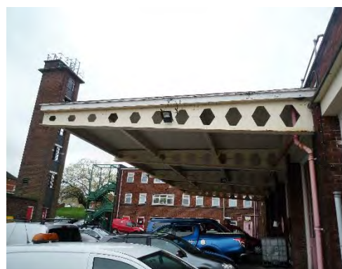
Figure 15. Overhang on Building 1 and fire tower within the centre of the site.
