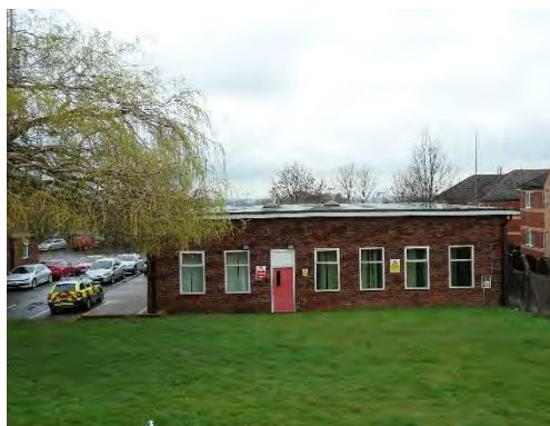
Figure 8. Southern aspect of Building 3 with intact windows and flat bitumen lined roof.
