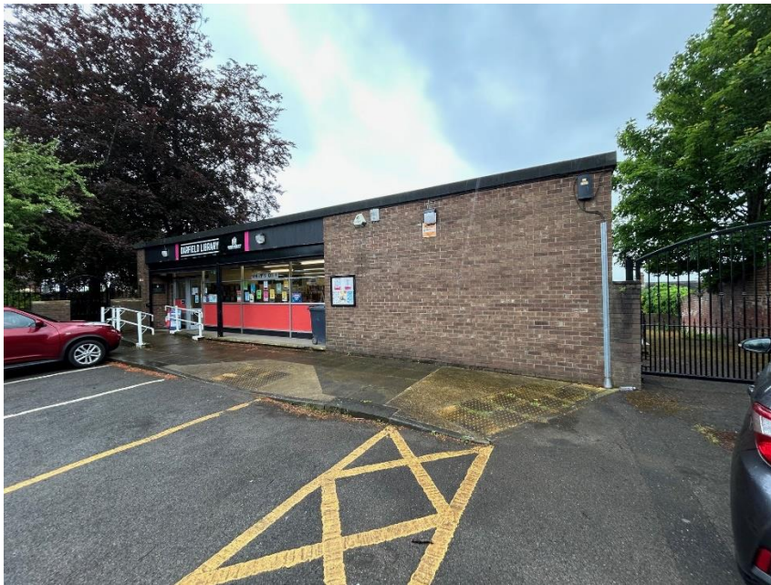
Photo of the existing Library building
