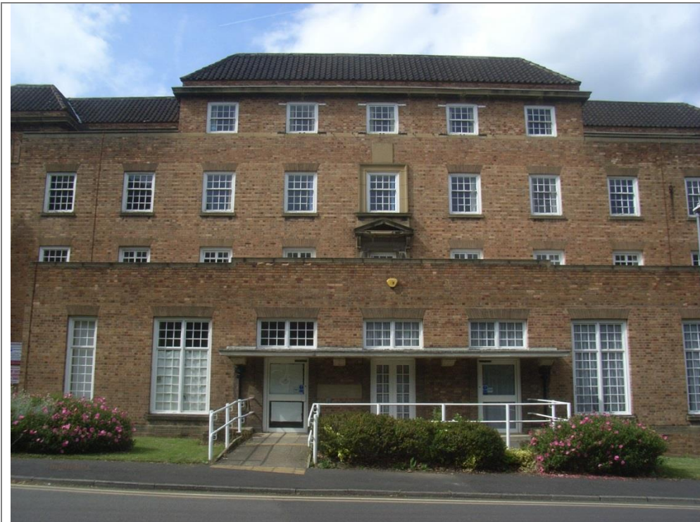
Plate 1: View to north from Berneslai Close of four storey building (TN2).
