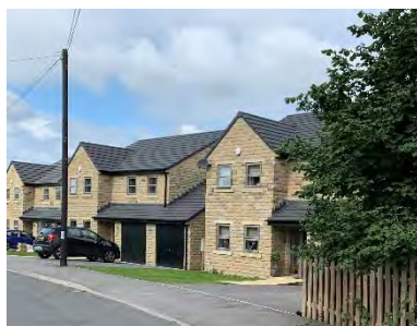
Adjacent new build properties
