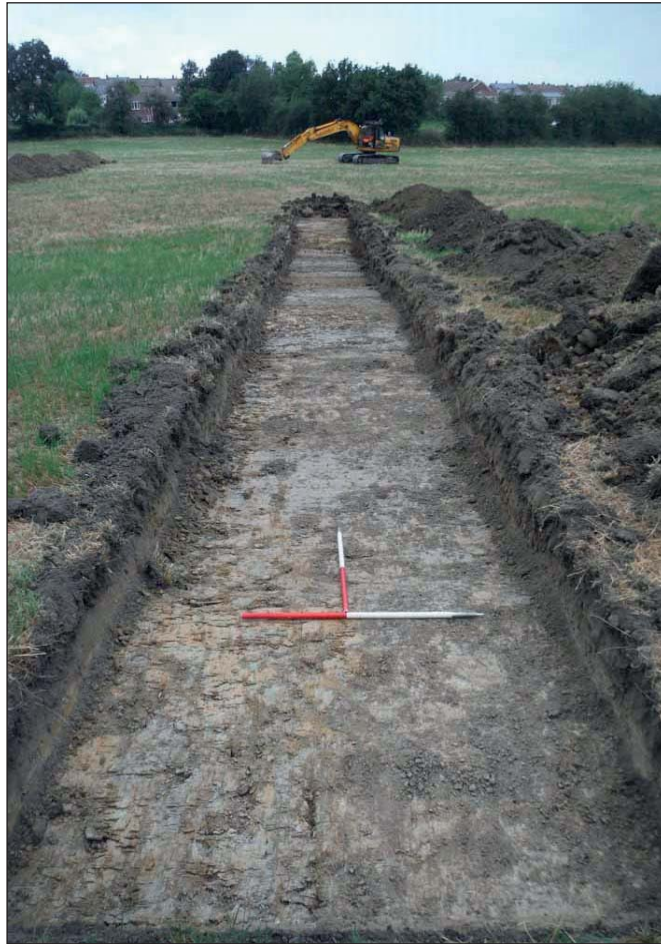
Plate 15. Trench 14, looking northeast
