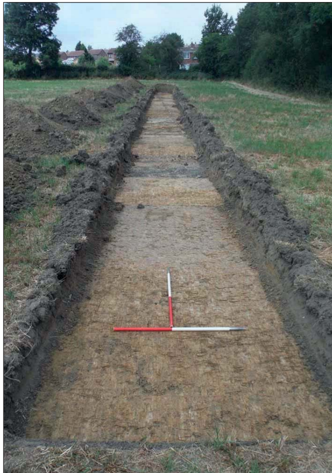
Plate 16. Trench 15, looking northwest
