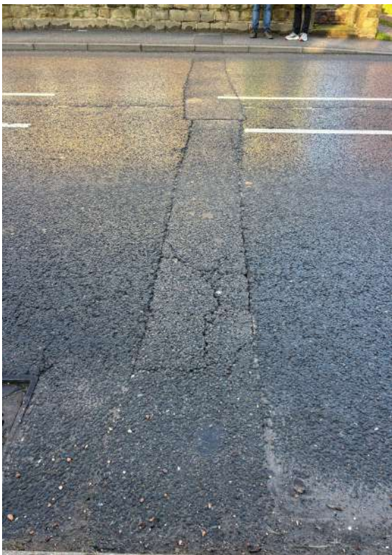
19 – Patchwork tarmac cracking and rutting.
