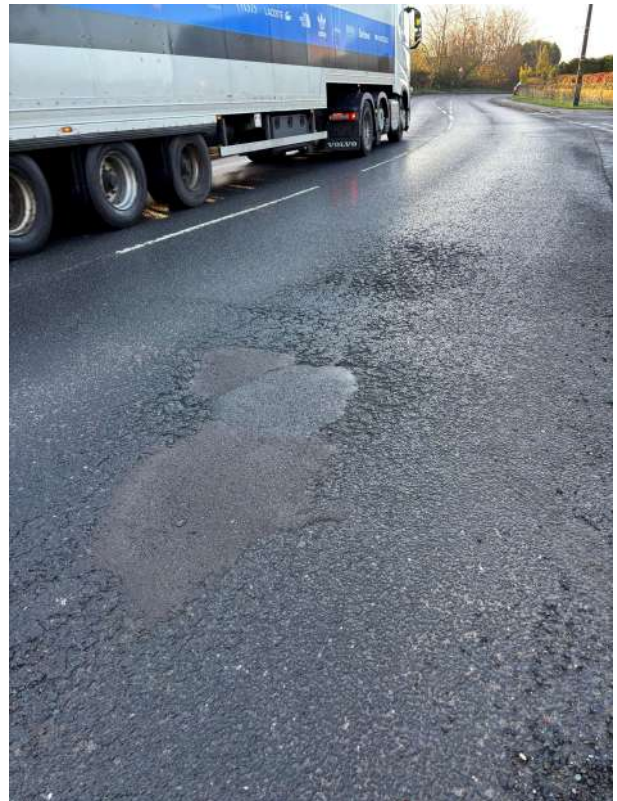
12 – Patchwork tarmac and crocodile cracking within highway.
