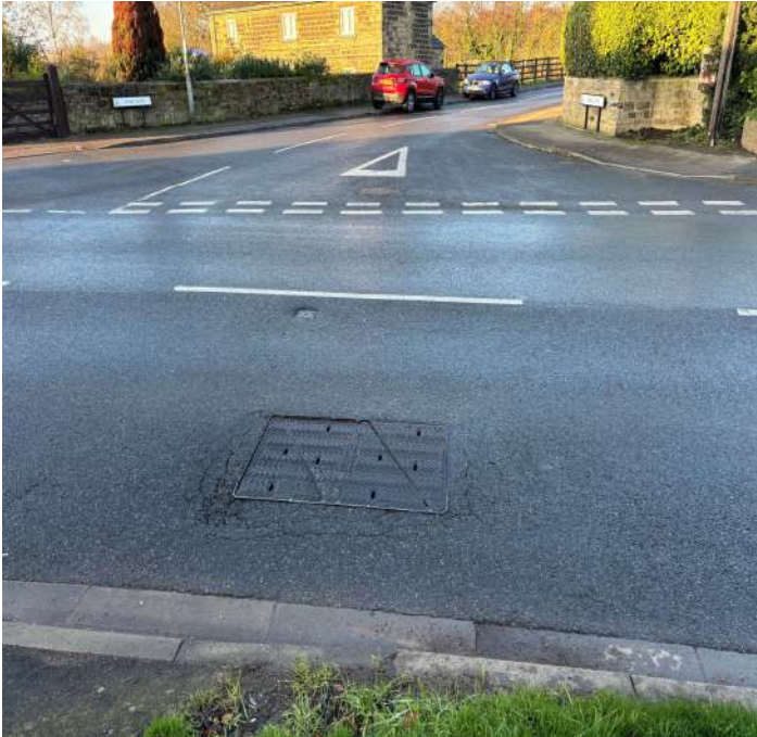
23 – Manhole in recently been patched and in good condition.
