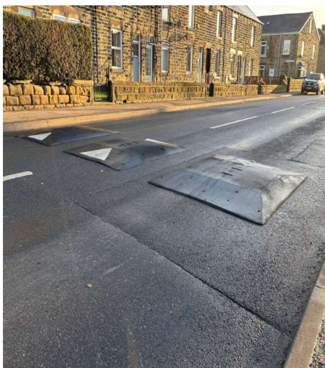
28 – Extents of highway, traffic calming measures (speed ramps).
