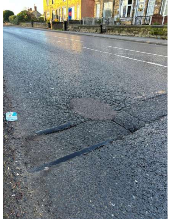
20 – Cracking in carriageway in junction outside entrance to park lane.
