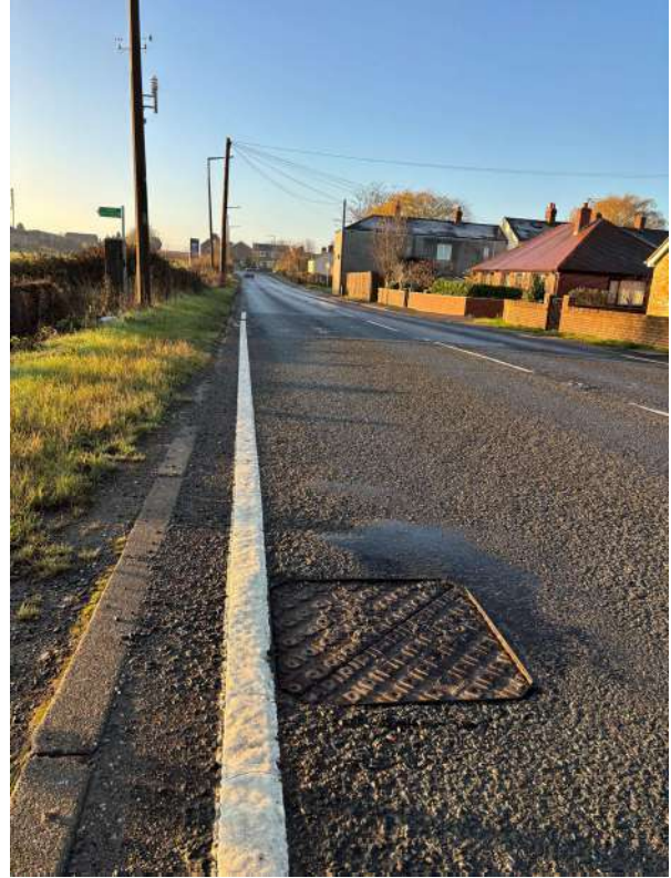
4 – Manhole cover to receive heavy traffic.
