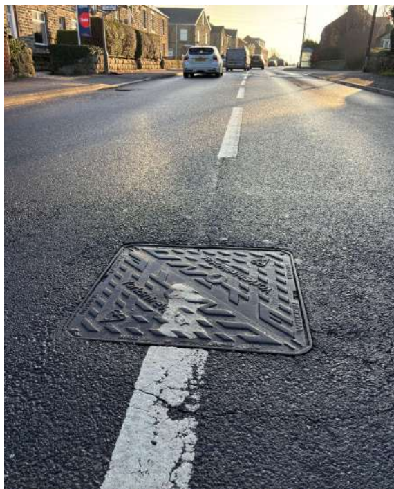
25 – Manhole which will receive heavy traffic in good condition.
