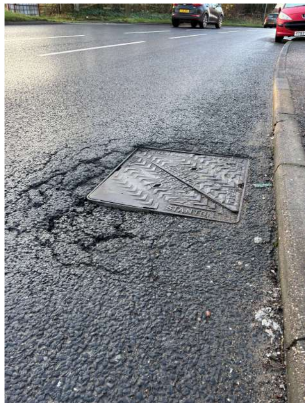
16 – Manhole cover in poor condition to receive heavy traffic.
