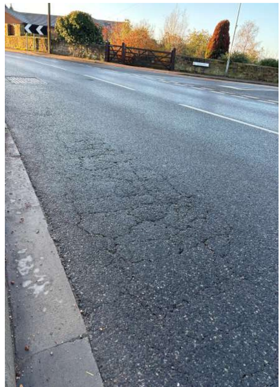
20 – Cracking in carriageway in junction outside entrance to park lane.
