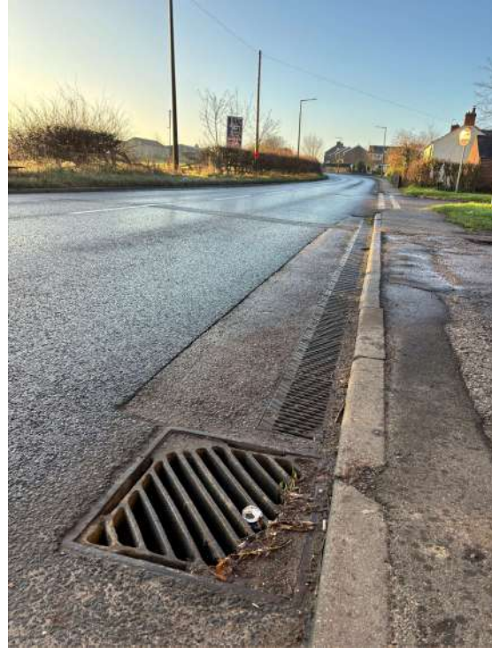
6 – Gully and ACO channel drain likely to suffer heavy HGV traffic.
