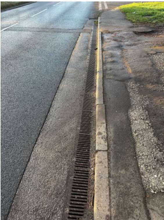
7 – Additional photo of ACO drain.
