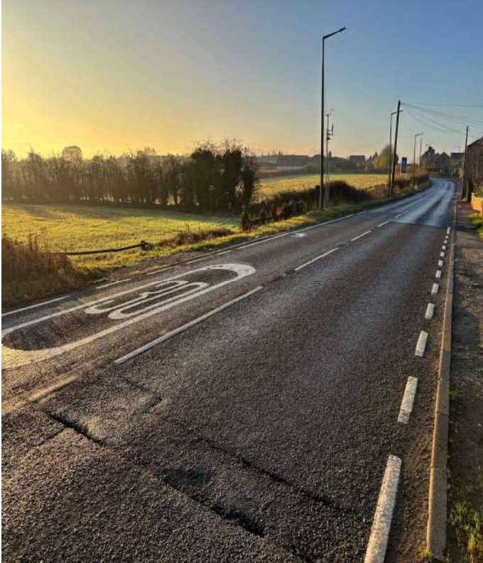
3 – Cracking and depression in carriageway.
