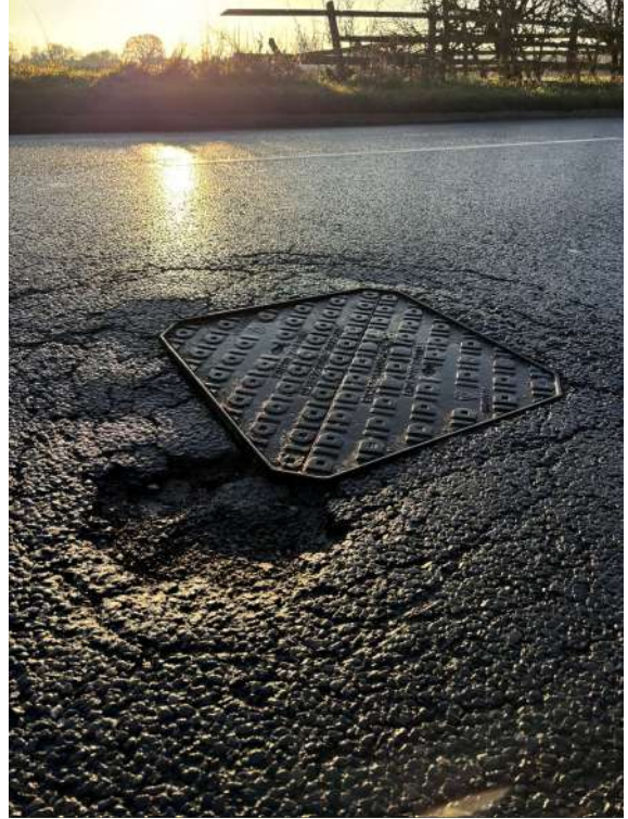
12 – Patchwork tarmac and crocodile cracking within highway.
