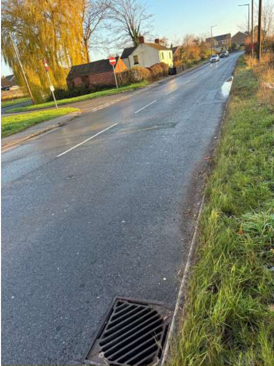
5 – Carriageway generally in good condition.
