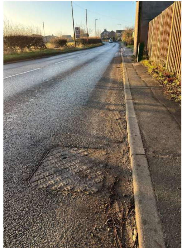
4 – Manhole cover to receive heavy traffic.
