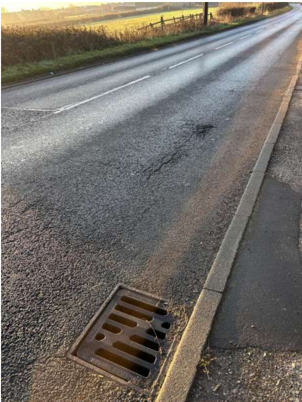
3 – Cracking and depression in carriageway.
