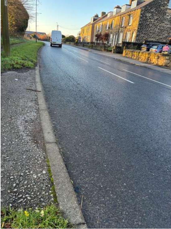
19 – Patchwork tarmac cracking and rutting.
