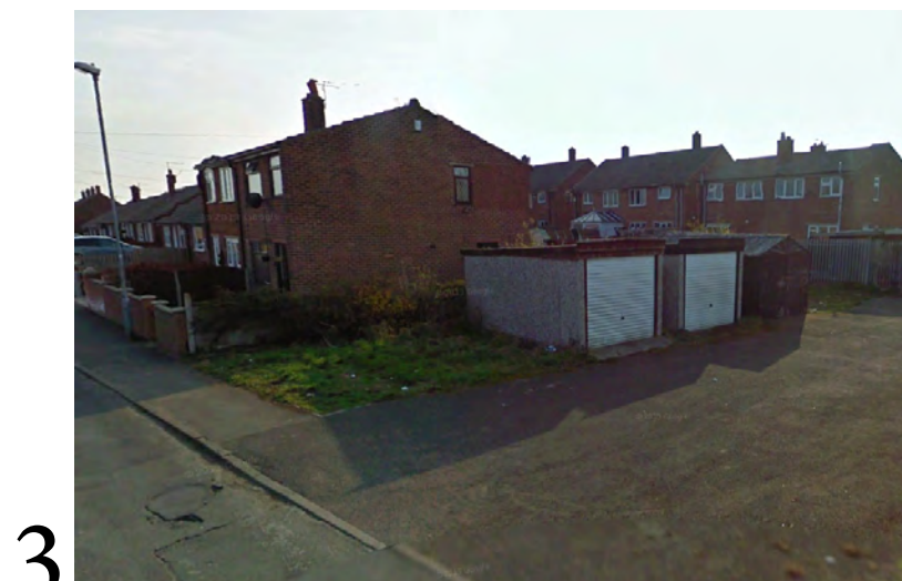
2 View of site from the South
