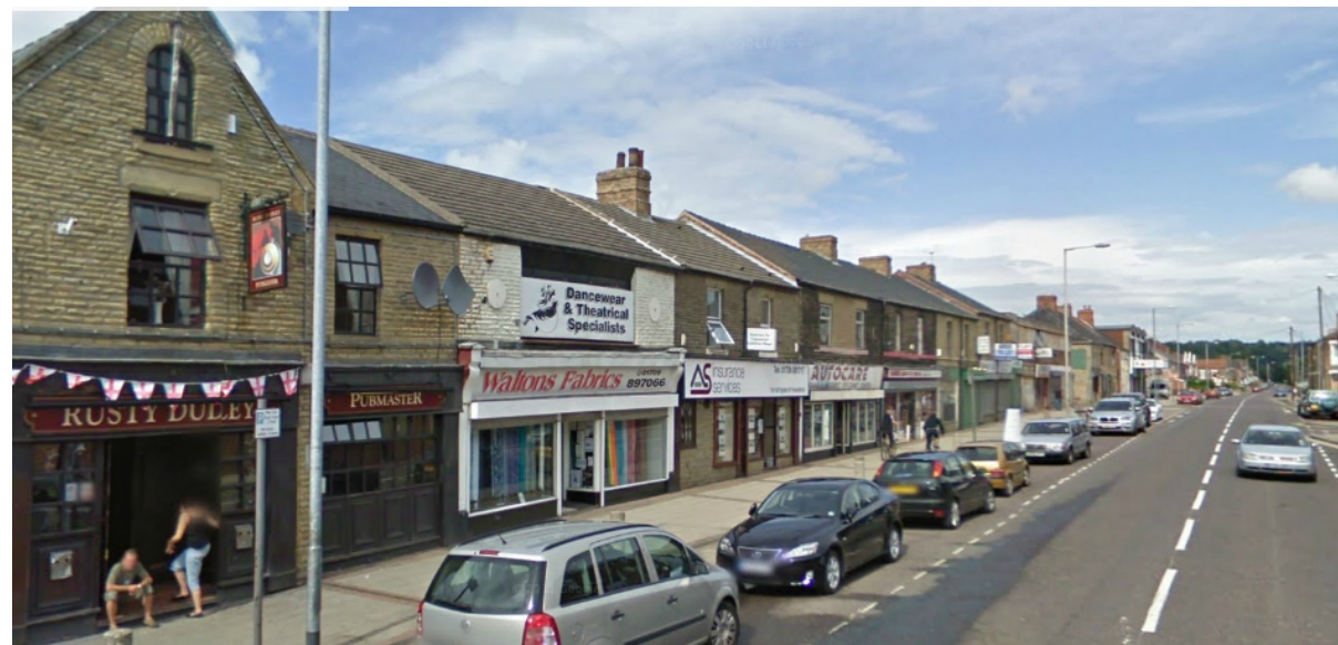
7. View east from along Doncaster Rd pre demolition.
