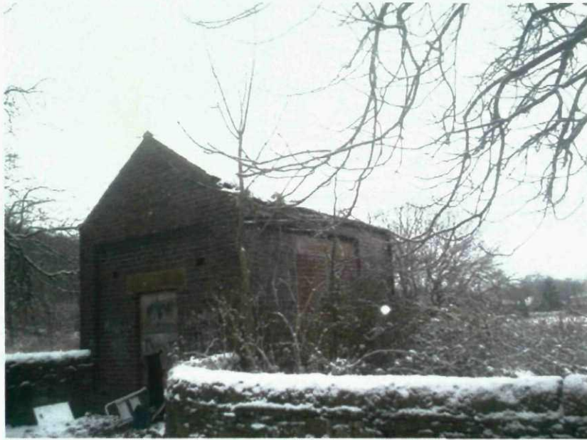
Structure with bat potential [above] at the Saunderson Road site.
