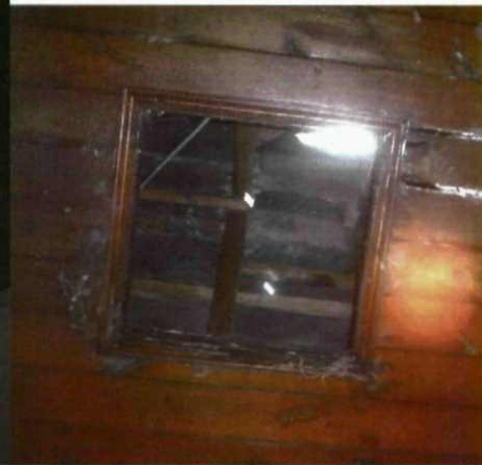
View from the loft into the roof Void which could not be properly inspected
