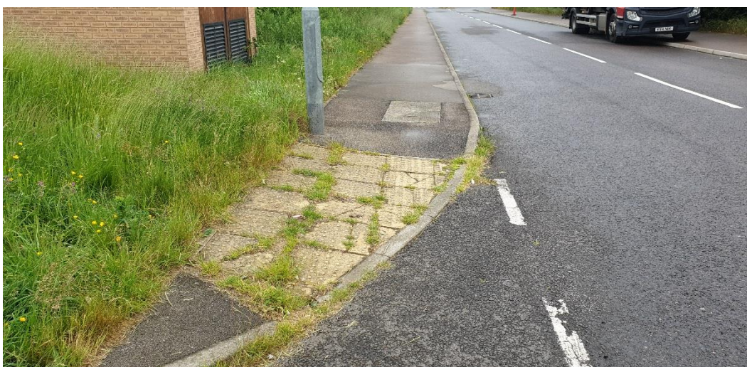
Figure 12 - Western side of entrance. Heavy vegetation in between tactile pavers.
