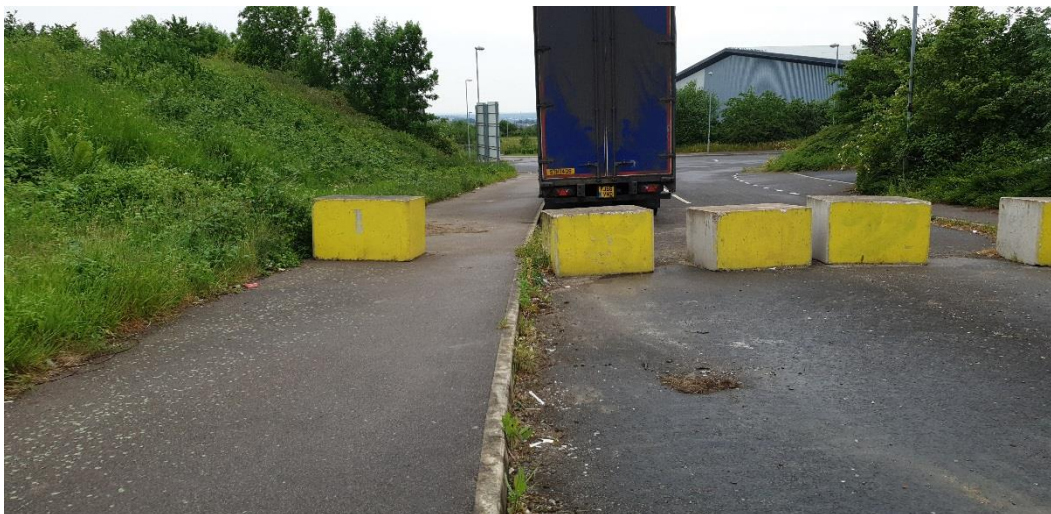
Figure 38 - Looking north through concrete blocks. Carriageway south of the blocks is not finished with surface course.
