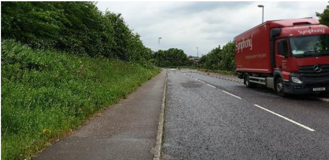
Figure 14 - View west of southern footway.
