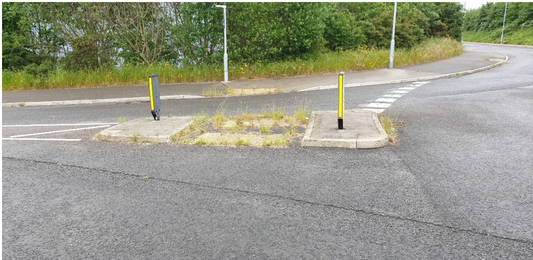
Figure 31 - Island on northern leg. Overgrown with weeds and vegetation etc.
