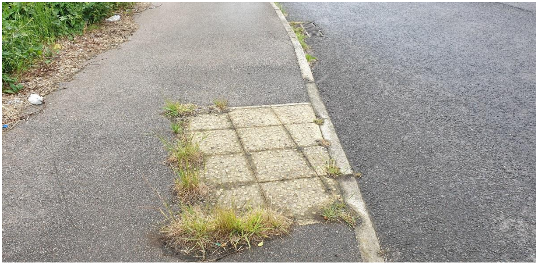
Figure 30 - West side of northern leg - tactile pavers.
