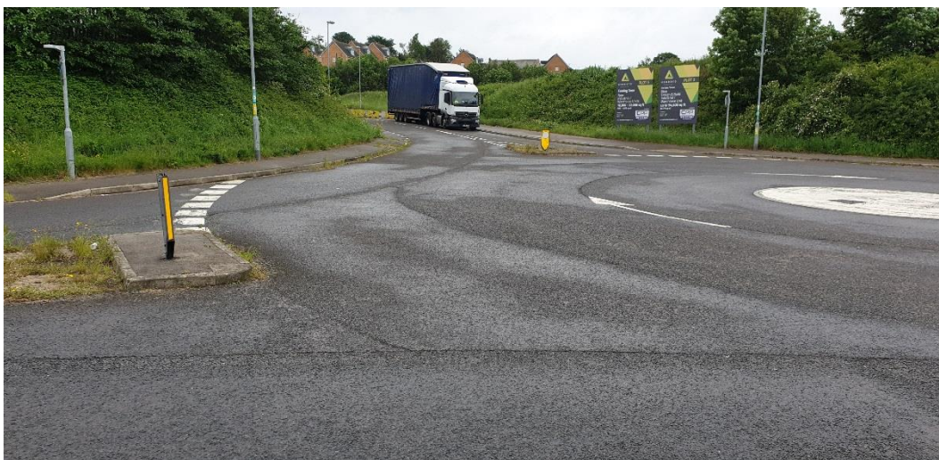
Figure 18 - View from northern side of eastern leg to the southern leg (Access to Plot 5)
