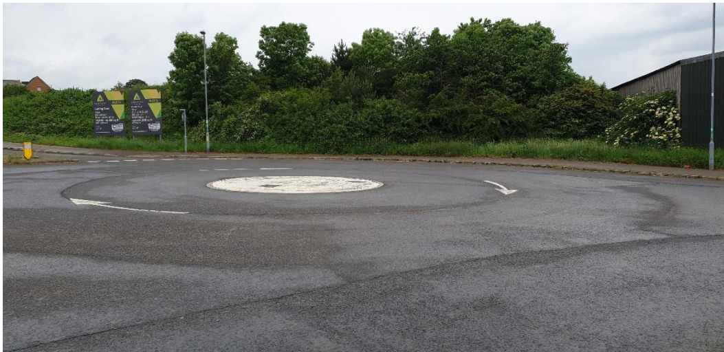
Figure 20 - View of surfacing across mini roundabout.
