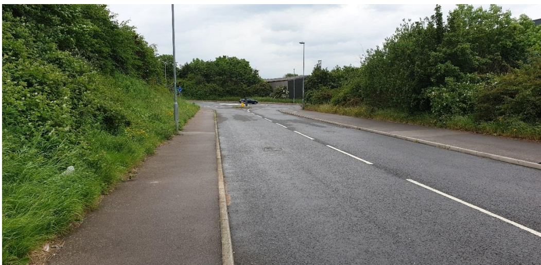
Figure 15 - View west on approach to mini roundabout.
