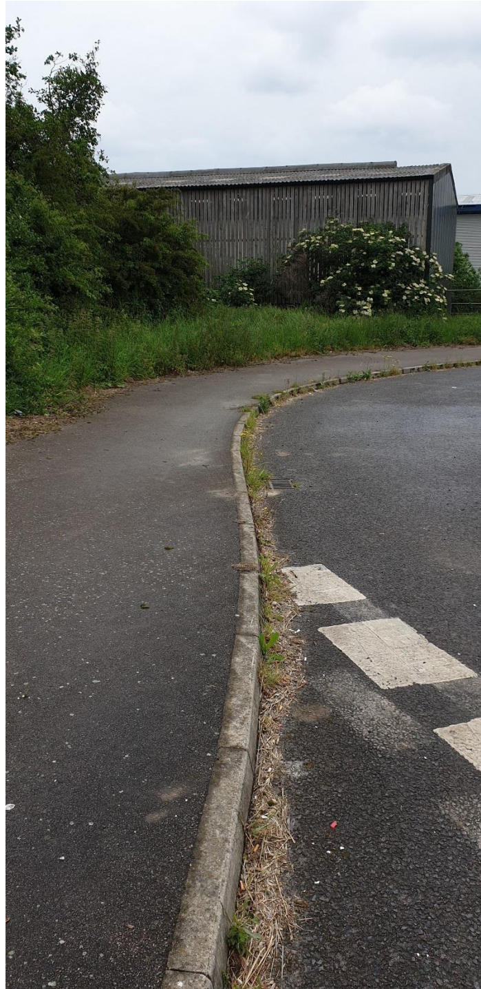
Figure 28 - Kerb line on western side of roundabout looking north from southern leg.
