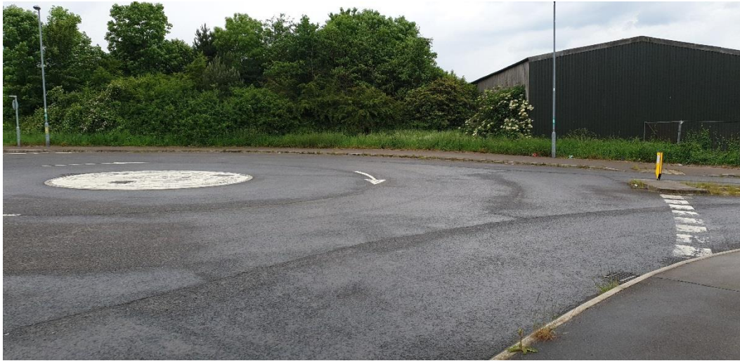
Figure 19 - View from eastern leg to northern leg.
