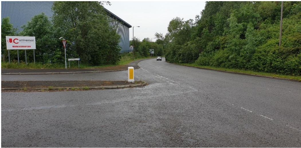
Figure 1 - View South across Junction with Ryecroft Bank.
