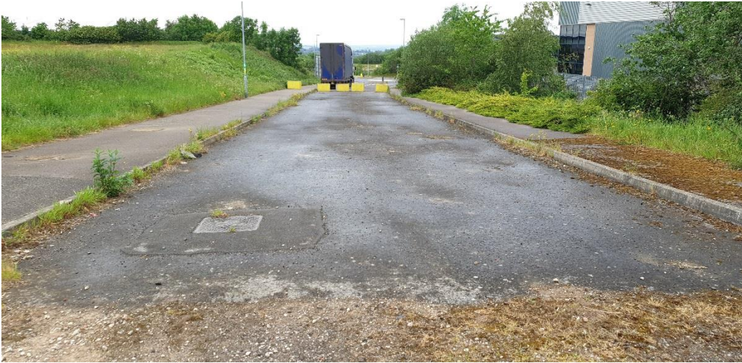
Figure 46 - View north from end of macadam binder course.
