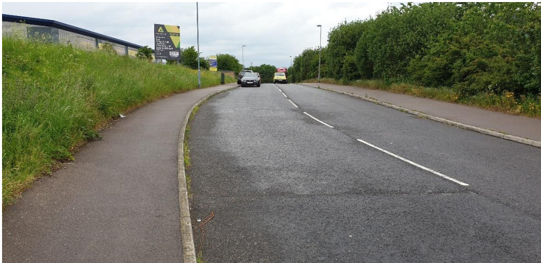
Figure 8 - Southern footway on Ashroyd Way looking west.
