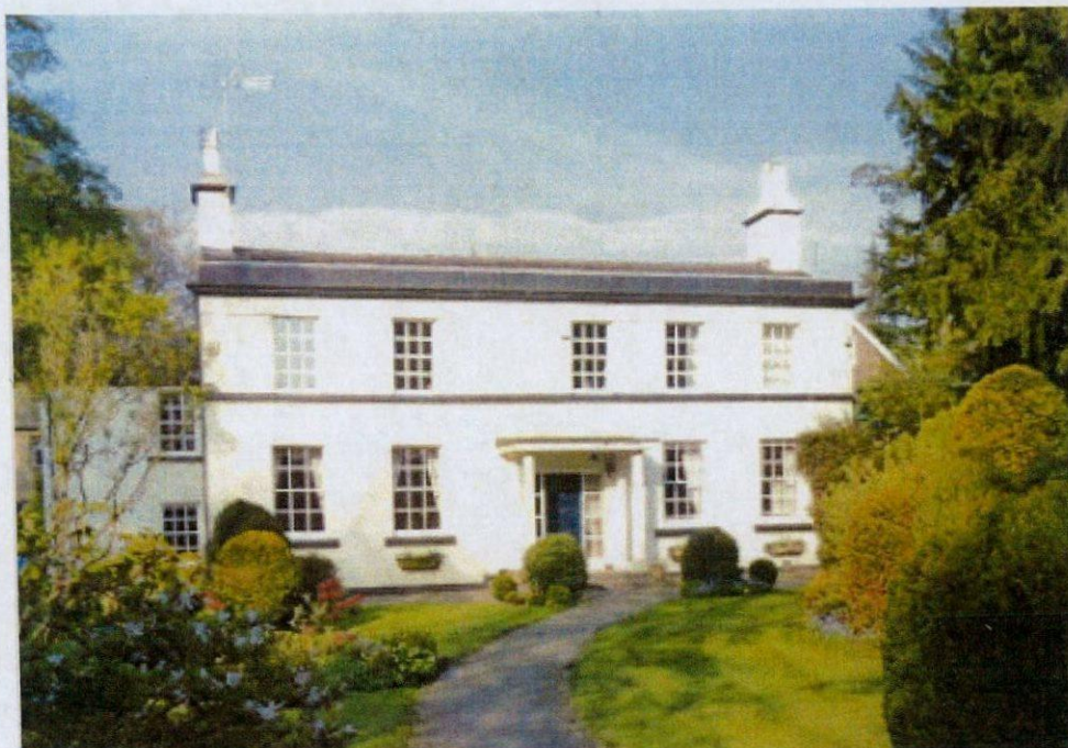
Fig 4 The former portico in position
