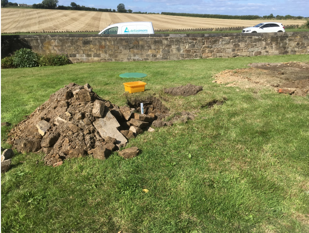
Photograph 5 – Position of FD101 (left of image) in relation to SA101 (top right of image). Demolition rubble excavated from FD101 can be seen stockpiled to the left of the hole. Facing approximately north.
