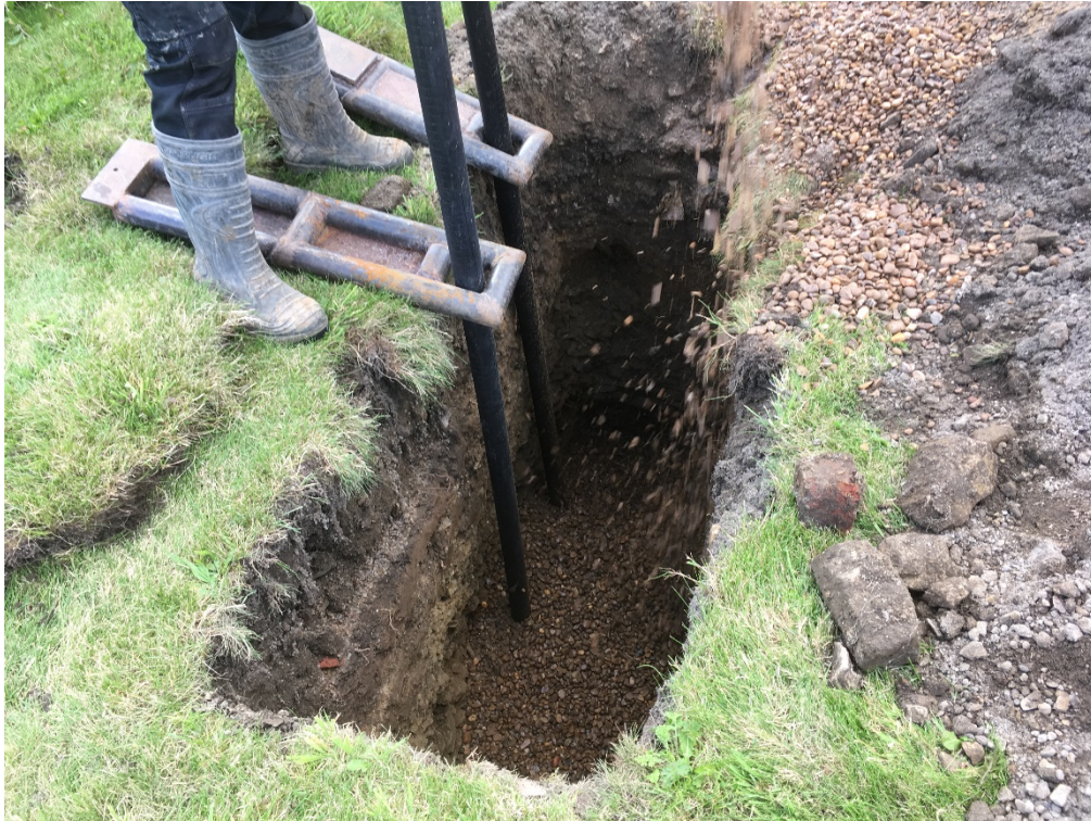
Photograph 3 – Soakaway installation in SA101. Pipework and gravel are being placed, with the gravel pack filling the trial pit from 2.3 to 1.5 m bgl.
