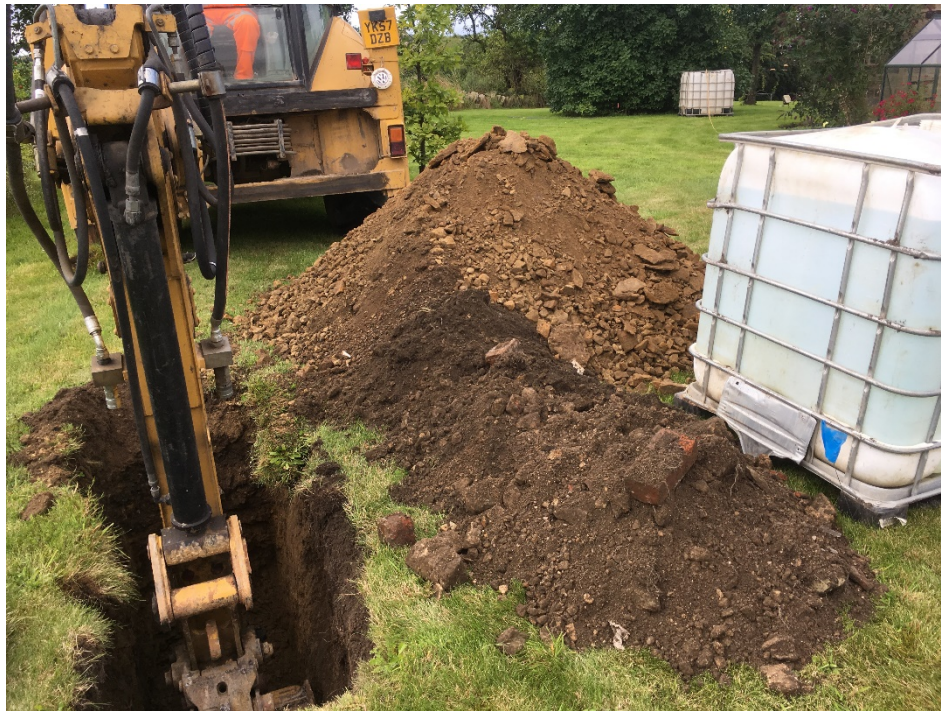
Photograph 1 – Excavation of SA101 to 2.3 m bgl. Facing approximately south.
