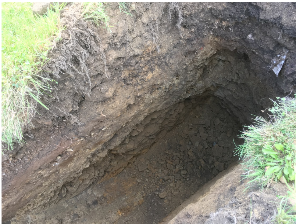
Photograph 2 – View at the base of SA101 (2.3 m bgl). Made Ground is present up to 0.65 m bgl, with weathered sandstone bedrock being encountered at 1.5 m bgl. Facing approximately south-east.
