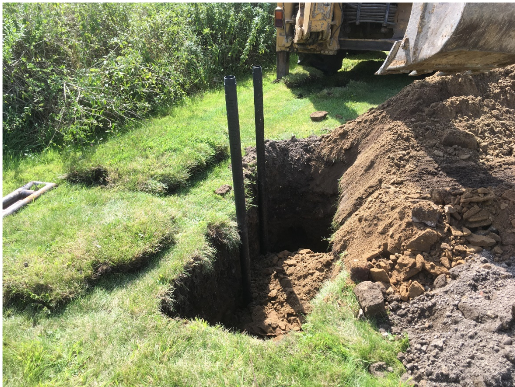
Photograph 4 – Backfilling of SA101 with arisings from 1.5 m bgl to ground level. Facing approximately south-east.
