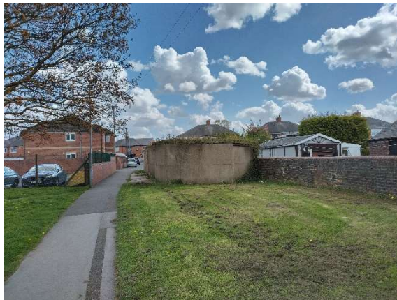
Photo 3: Site from northwest
