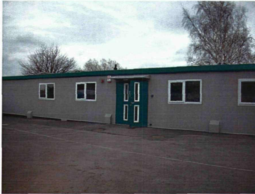
Image 1: Springwell modular building – Barnsley College propose to relocate the building for use on the Honeywell site.
