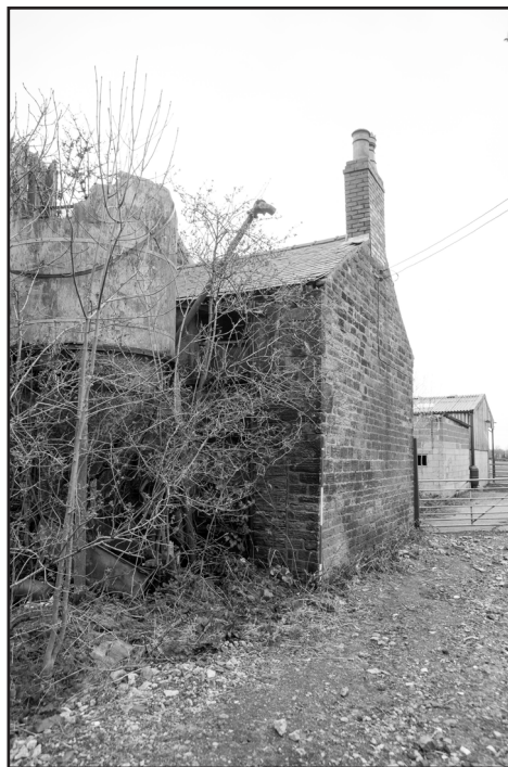
Photograph Number: 12 Reference: RLHS_012 Description: Gable end to Cottage 1 Direction: NW
