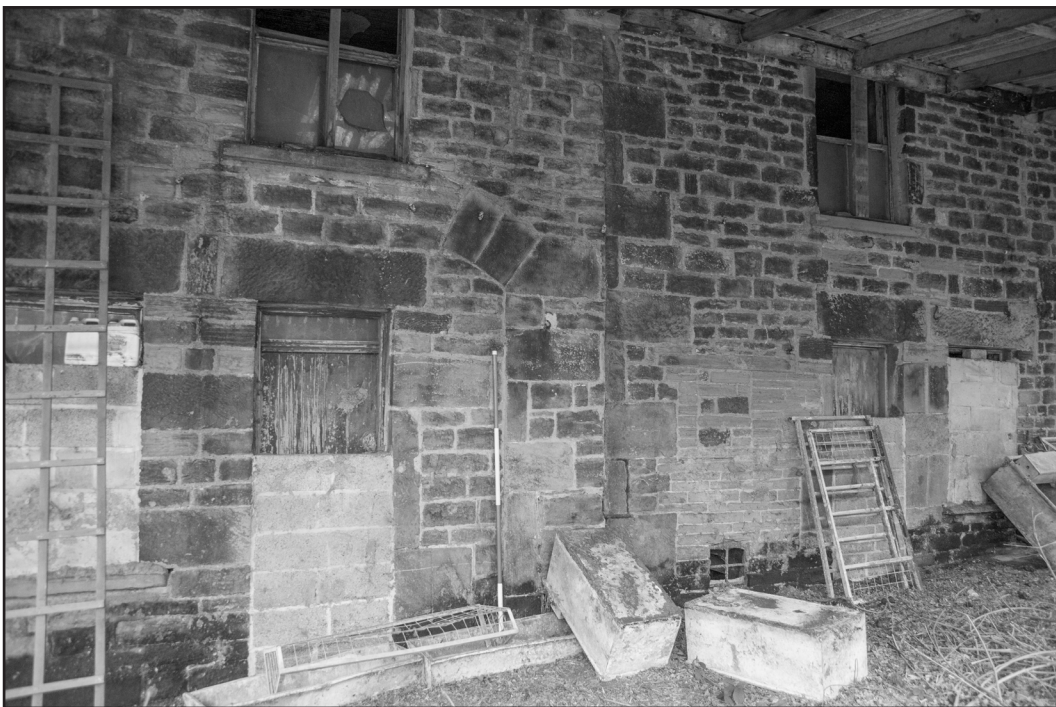
Photograph Number: 32 Reference: RLHS_032 Description: West elevation of the cottages showing a blocked former cart entry and a quoined straight joint Direction: S
