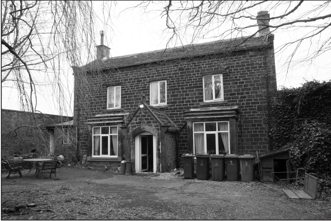
Photograph Number: 1 Reference: RLHS_001 Description: Front elevation of Roughbirchworth Lodge Direction: NW
