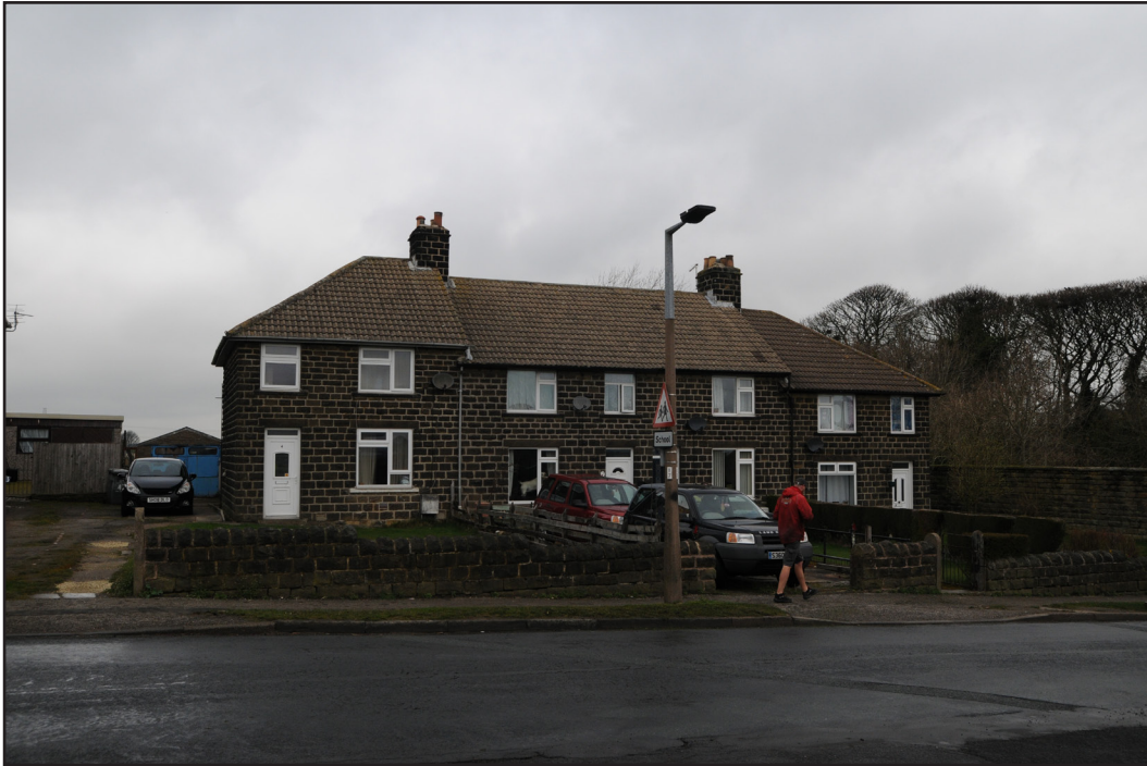
Photograph Number: 39 Description: Mid 20th-century housing along Roughbitchworth Lane Direction: NW
