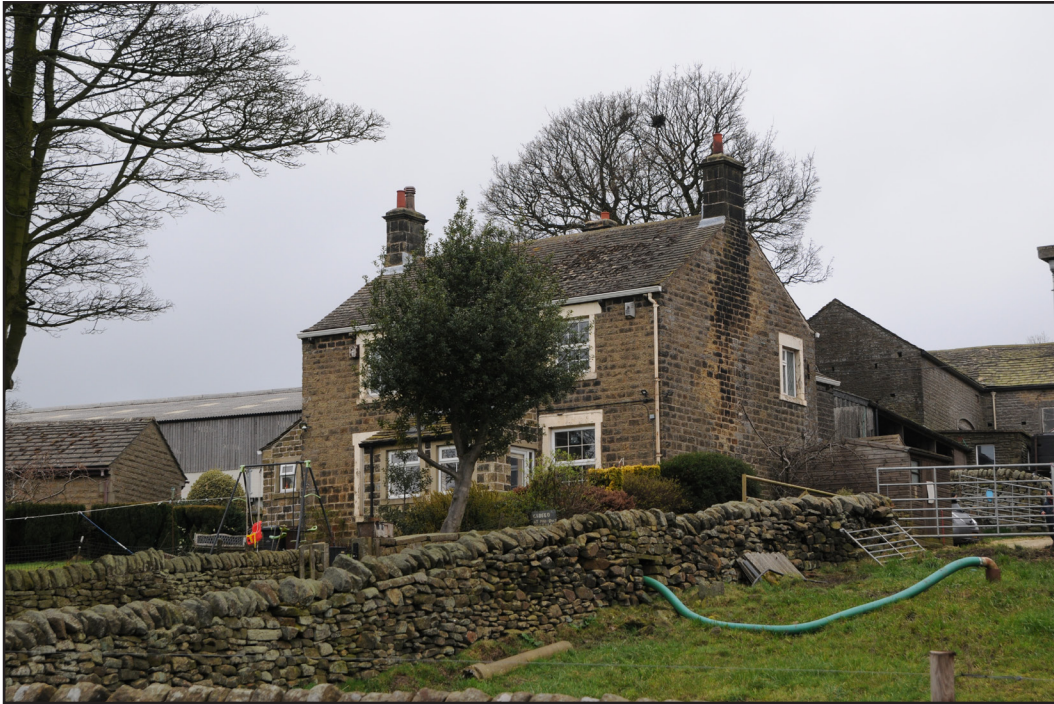
Photograph Number: 37 Sycamore House Direction: NW
