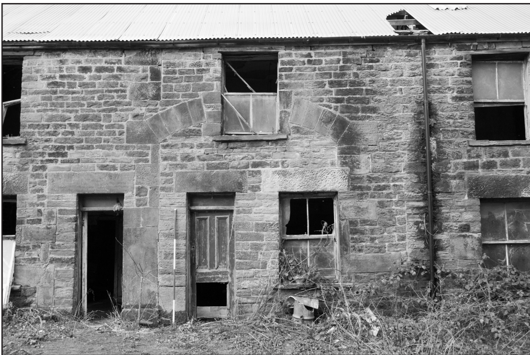
Photograph Number: 14 Reference: RLHS_014 Description: Blocked segmental-arched cart entry Direction: NW
