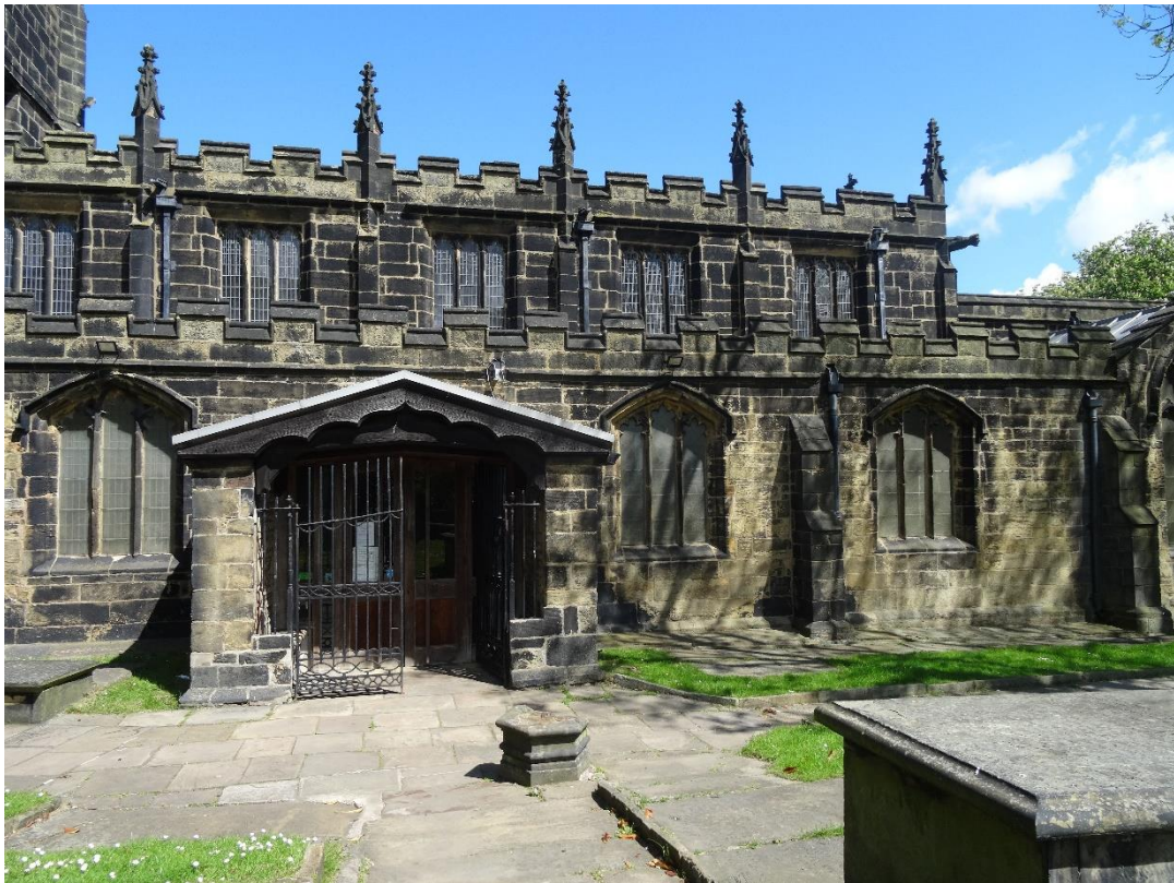
Nave roof is hidden by the parapet walls to all sides.
