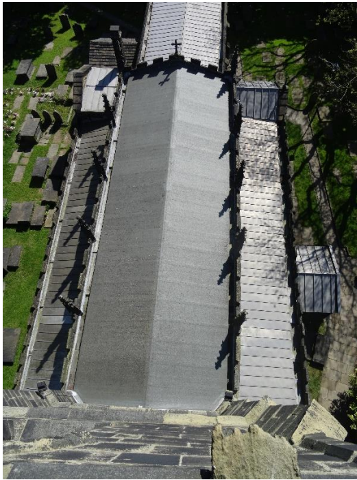
Nave roof viewed from the Tower
