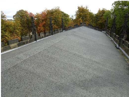
Felt roof covering to the Nave
