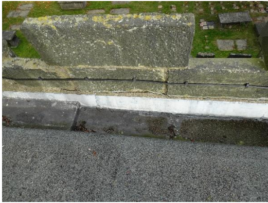
Lead gutters and outlets remain in place.
