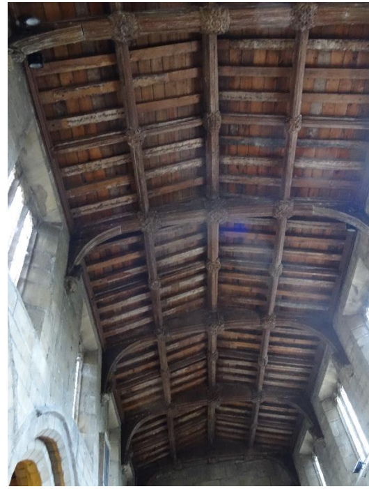
Exposed Nave roof structure (14 th Century)
