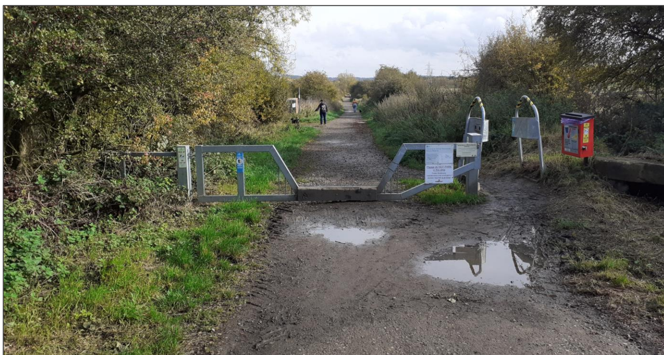
Plate 1: View of Lowfield Lane (looking east) a short distance to the north-east of the Site boundary
