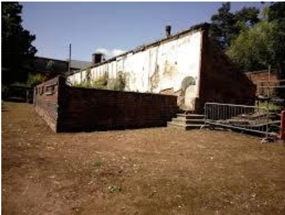
SOUTH EAST VIEW PRIOR TO REPAIR OF GLASSHOUSE TERRACES
