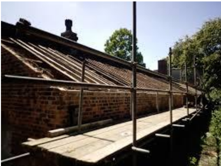
NORTH EAST VIEW OF ROOF UNDER RECENT REPAIR
