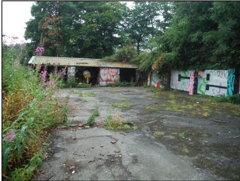
Figure 6. Hard standing and buildings on site.
