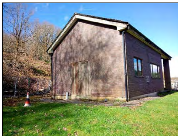
Photograph 14: Southeast corner of Building B5
