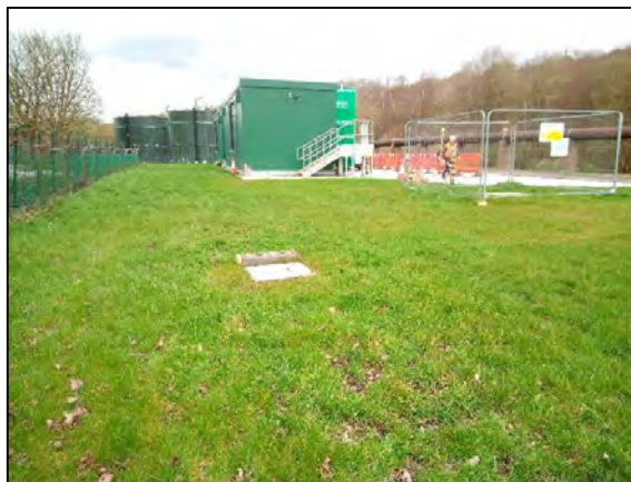
Photograph 2: Location of proposed ferric dosing kiosk, northern section of the site
