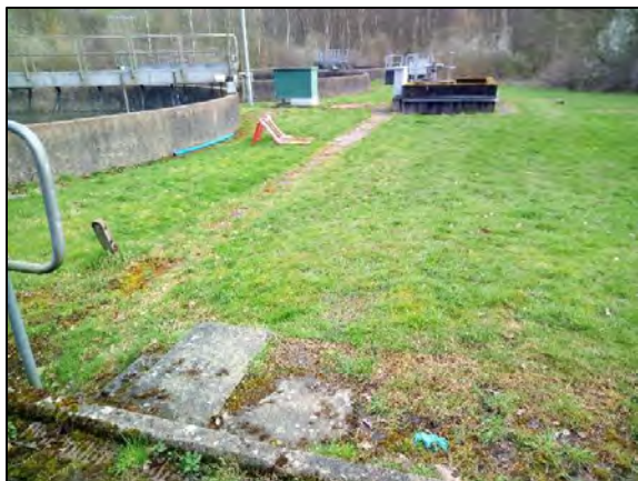
Photograph 1: Location of the proposed TSR pump station, southern section of the site
