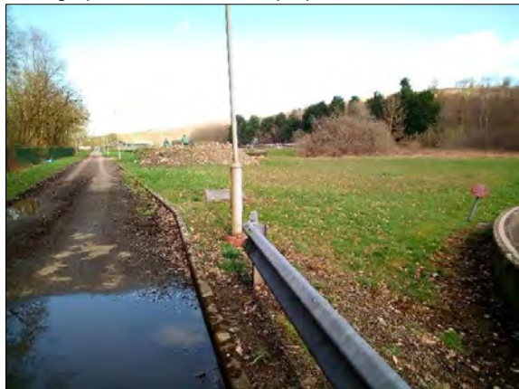
Photograph 3: Location of the proposed MCC kiosk
