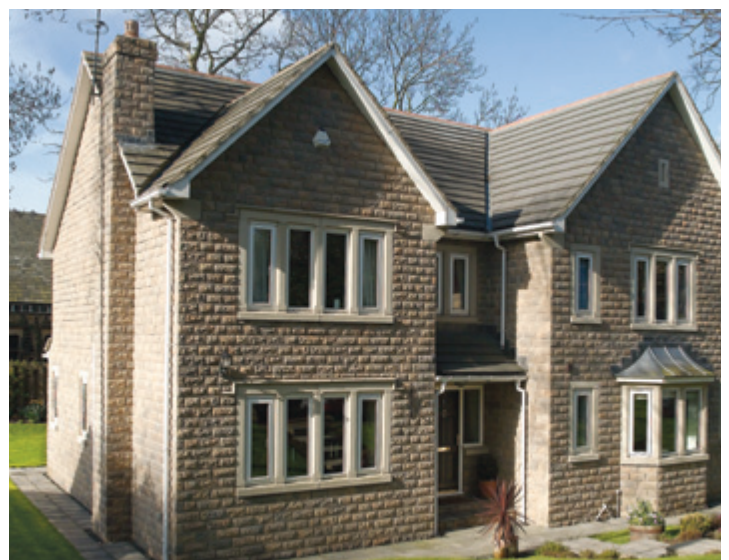
Heritage Sharp Face, Weathered Sandstone
