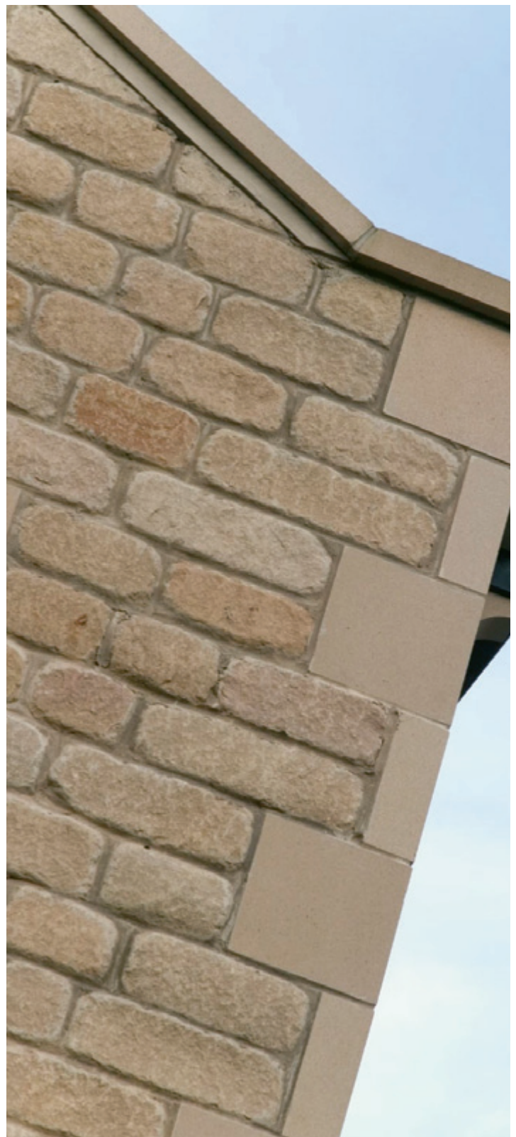
Cottage Walling detail at Sunnybank Mills, Meltham, Huddersfield
