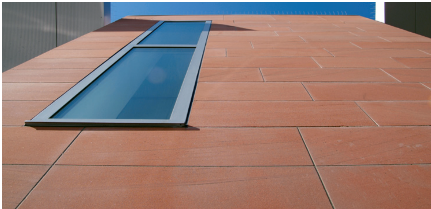
Rubbed Face Walling, Primark, Ayr Central
