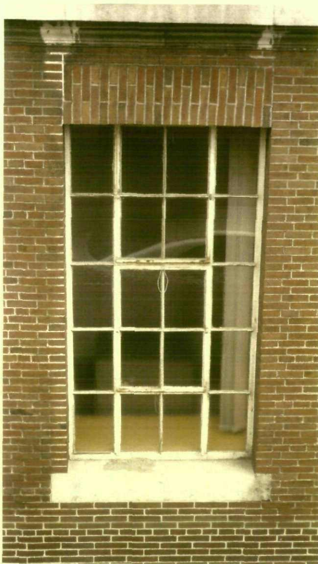
Window type 04 Proposal - To be replaced 2445 x 1300mm
