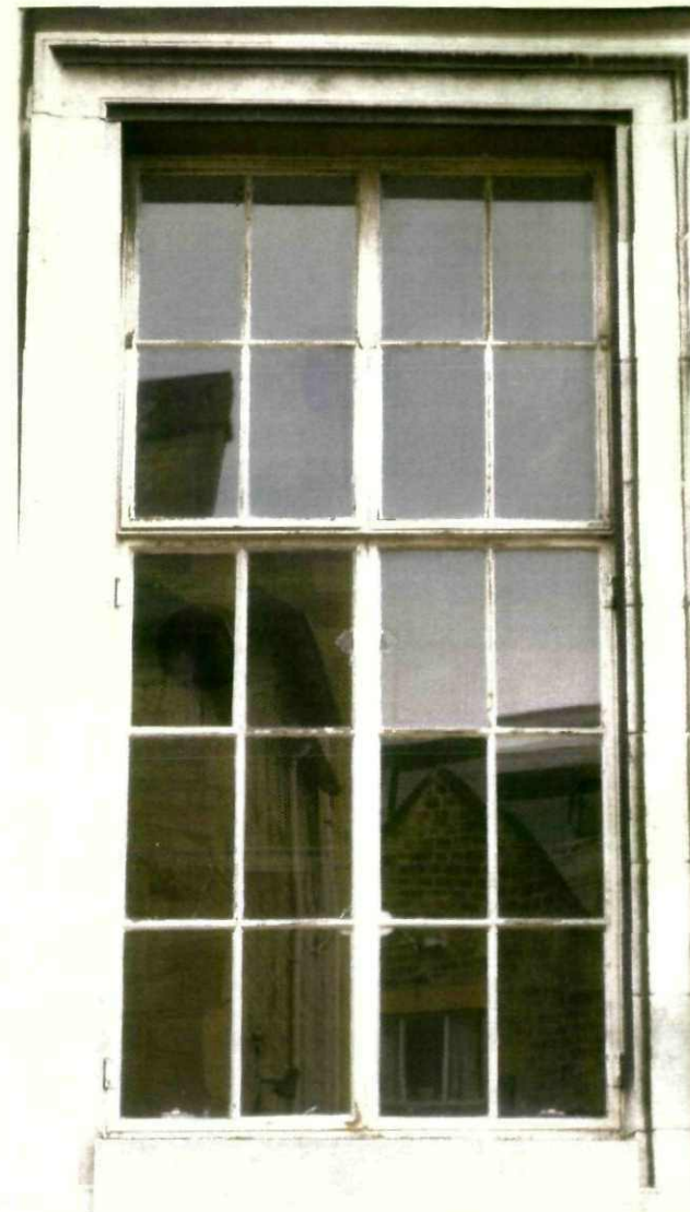
Window type 08 Proposal - To be replaced 2575 x 1300mm
