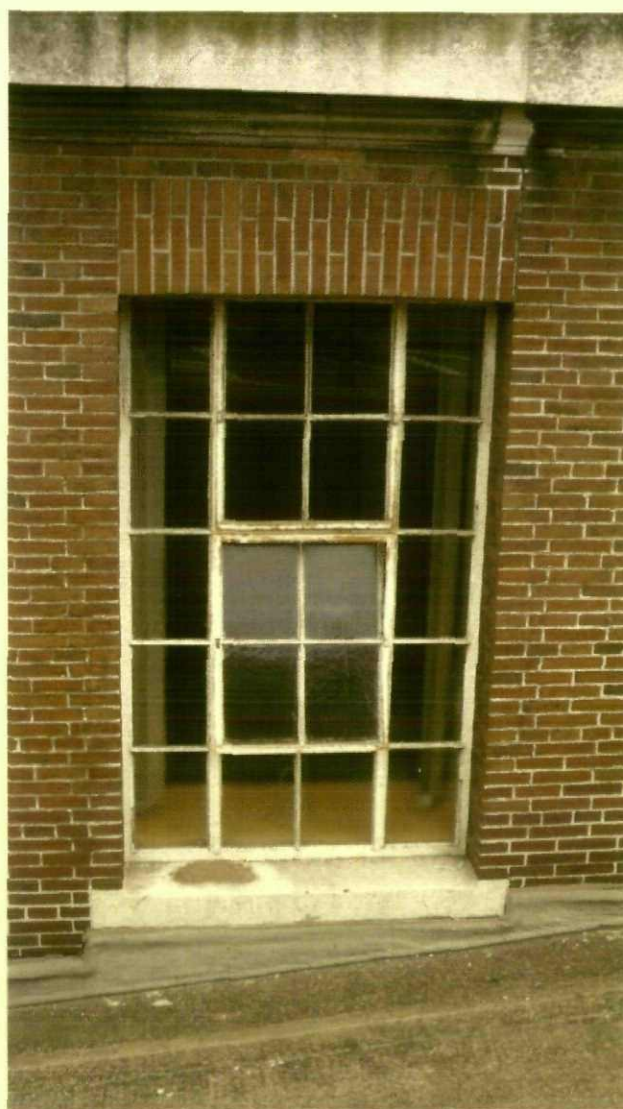
Window type 05 Proposal - To be replaced 2160 x 1300mm
