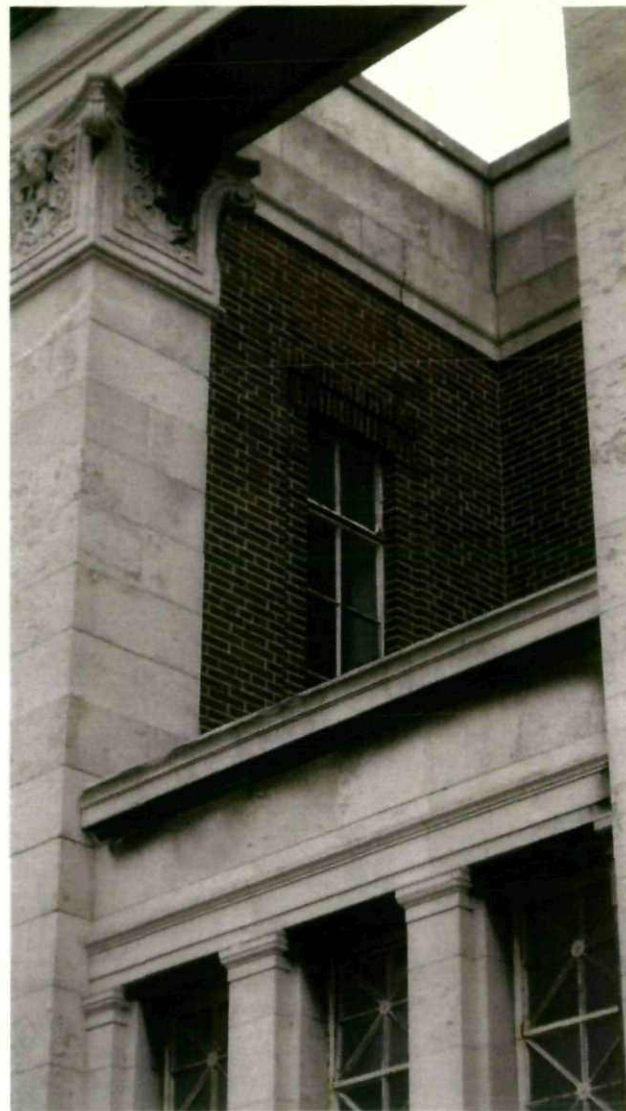
Window type 13 Proposal - To be replaced 1670 x 720mm
