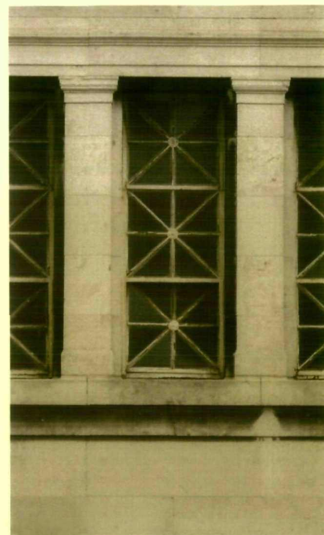
Window type 11 Proposal - To be refurbished 1600 x 550mm 3No per location
