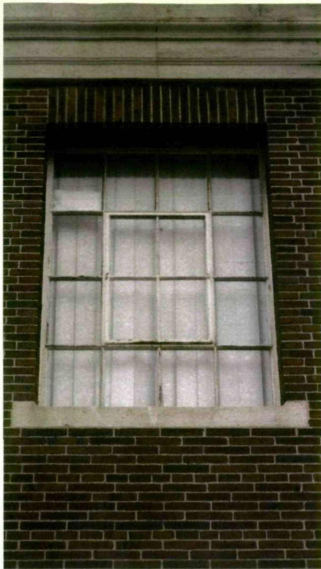
Window type 12 Proposal - To be replaced 2010 x 1300mm Identical to type 01
