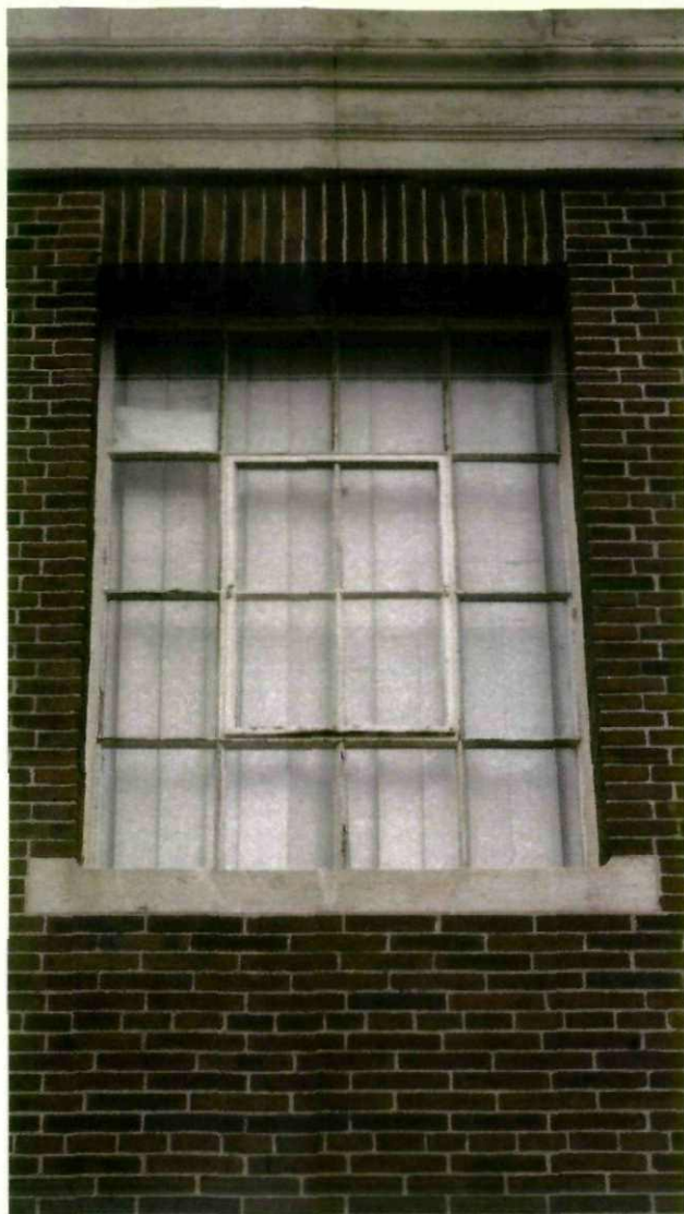
Window type 01 Proposal - To be replaced 2010 x 1300mm
