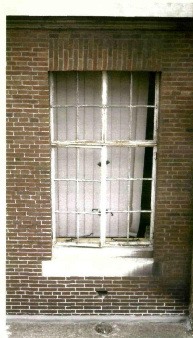
Window type 03 Proposal - To be replaced 2340 x 1300mm
