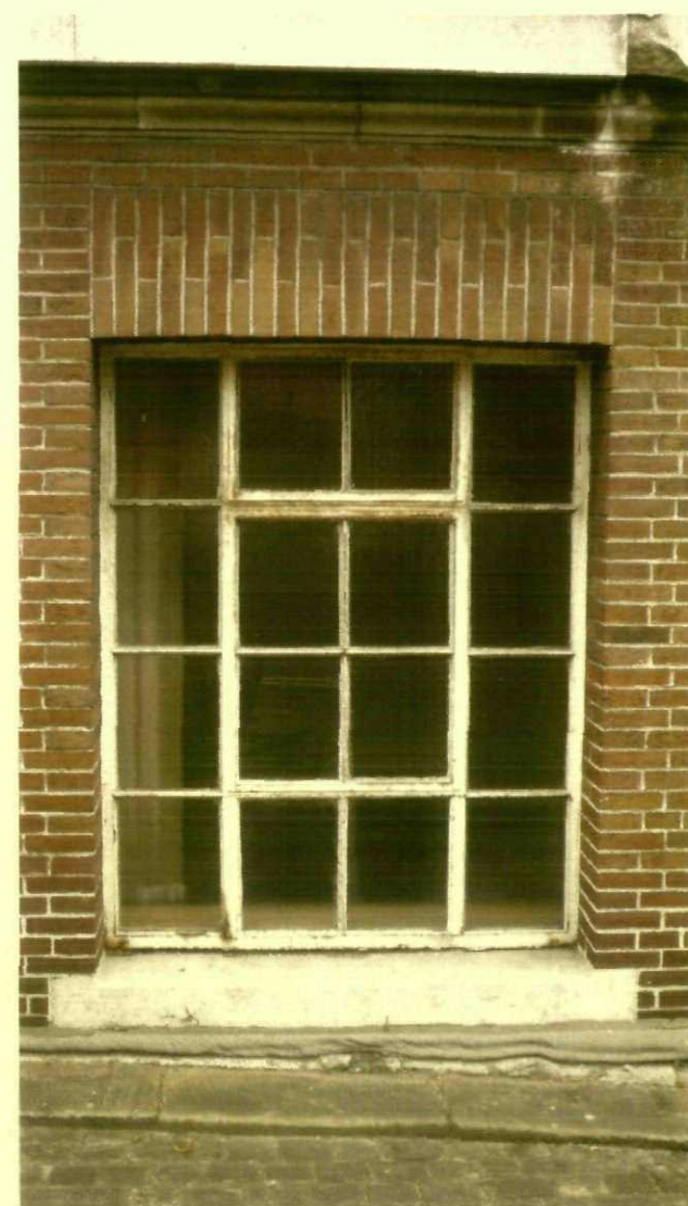
Window type 06 Proposal - To be replaced 1670 x 1300mm
