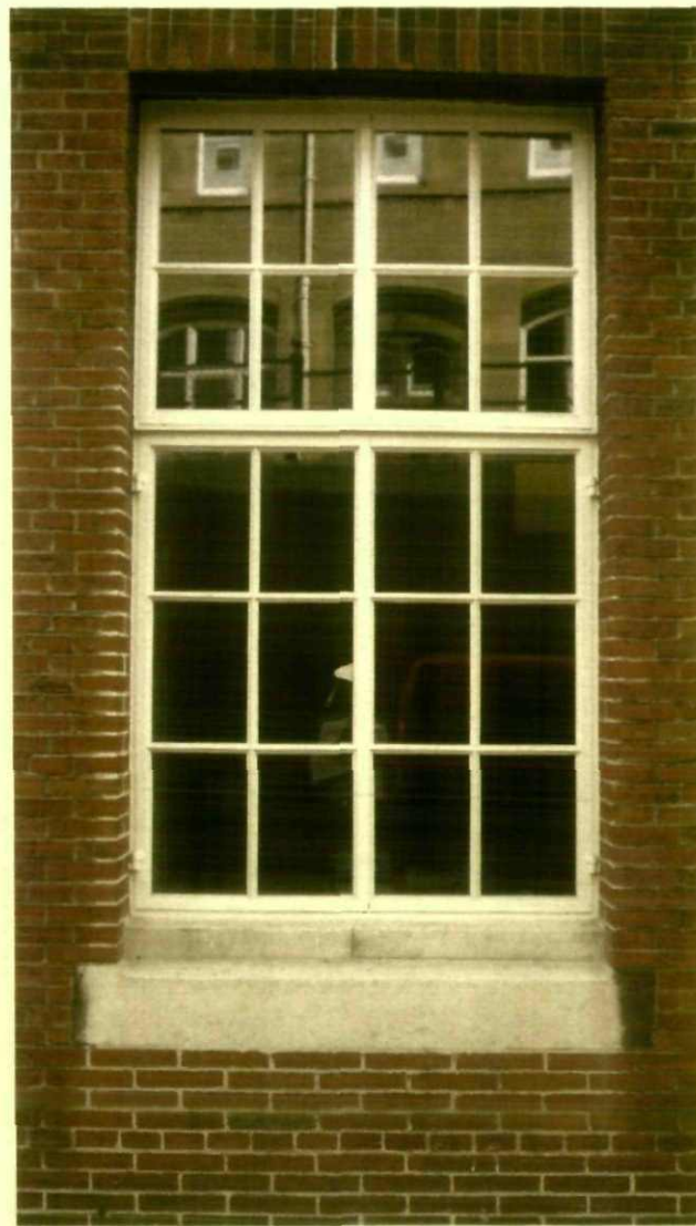
Window type 03 - ground floor typical Picture showing installed prototype W20 profiles with external silicone beading to double glazed units. 2340 x 1300mm
