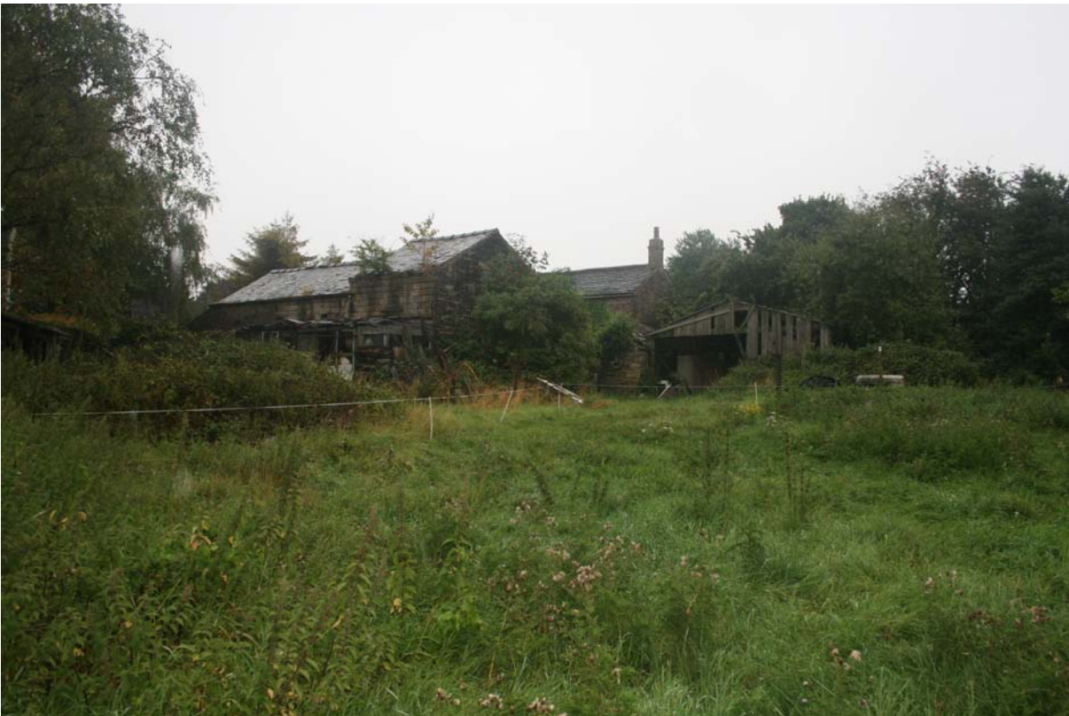
Plate 4. Farm buildings in southwestern boundary of site, looking S. The stone buildings will be unaffected by the proposed development although the timber lean-to will be demolished
