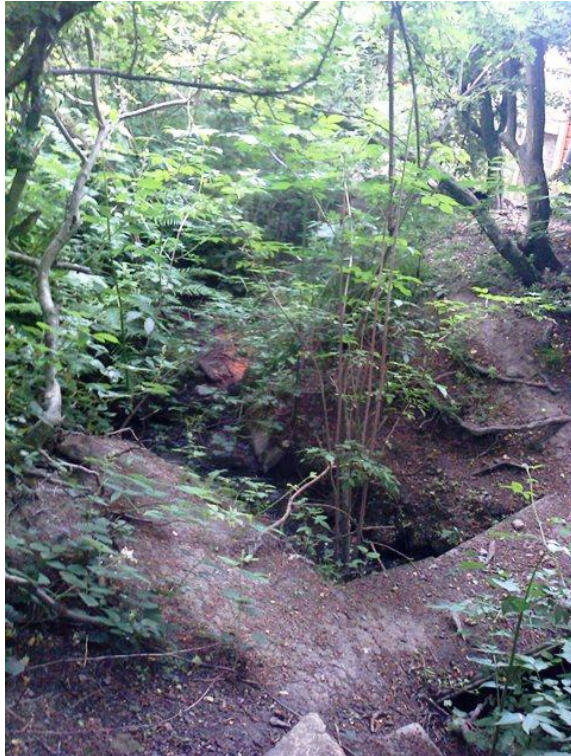
Photo 7. Section of drain near TN1, Figure 1
