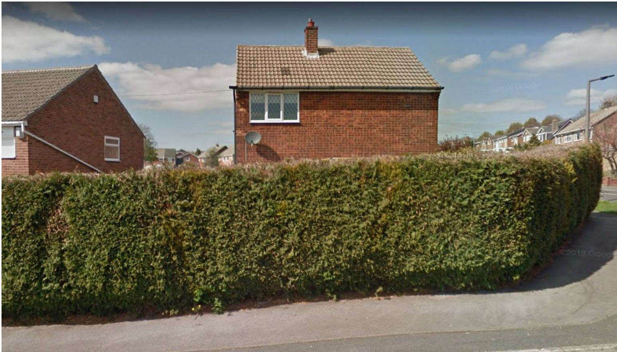
Existing rear view from Warwick Road.
