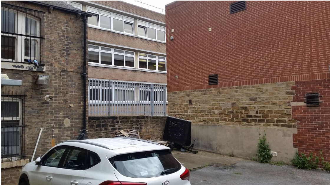
Picture 7:Rear of 7 Eastgate. It is an enclosed yard with no through traffic.
