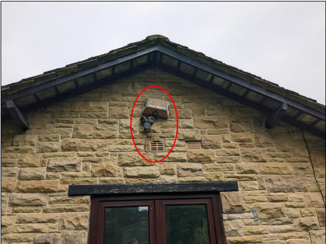
Plate 5. Air brick and alarm box on southwest gable
