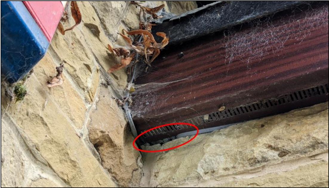
Plate 5. Air brick and alarm box on southwest gable
