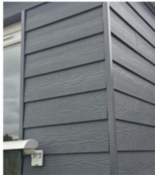
Dormer walls grey PVCu weatherboard
