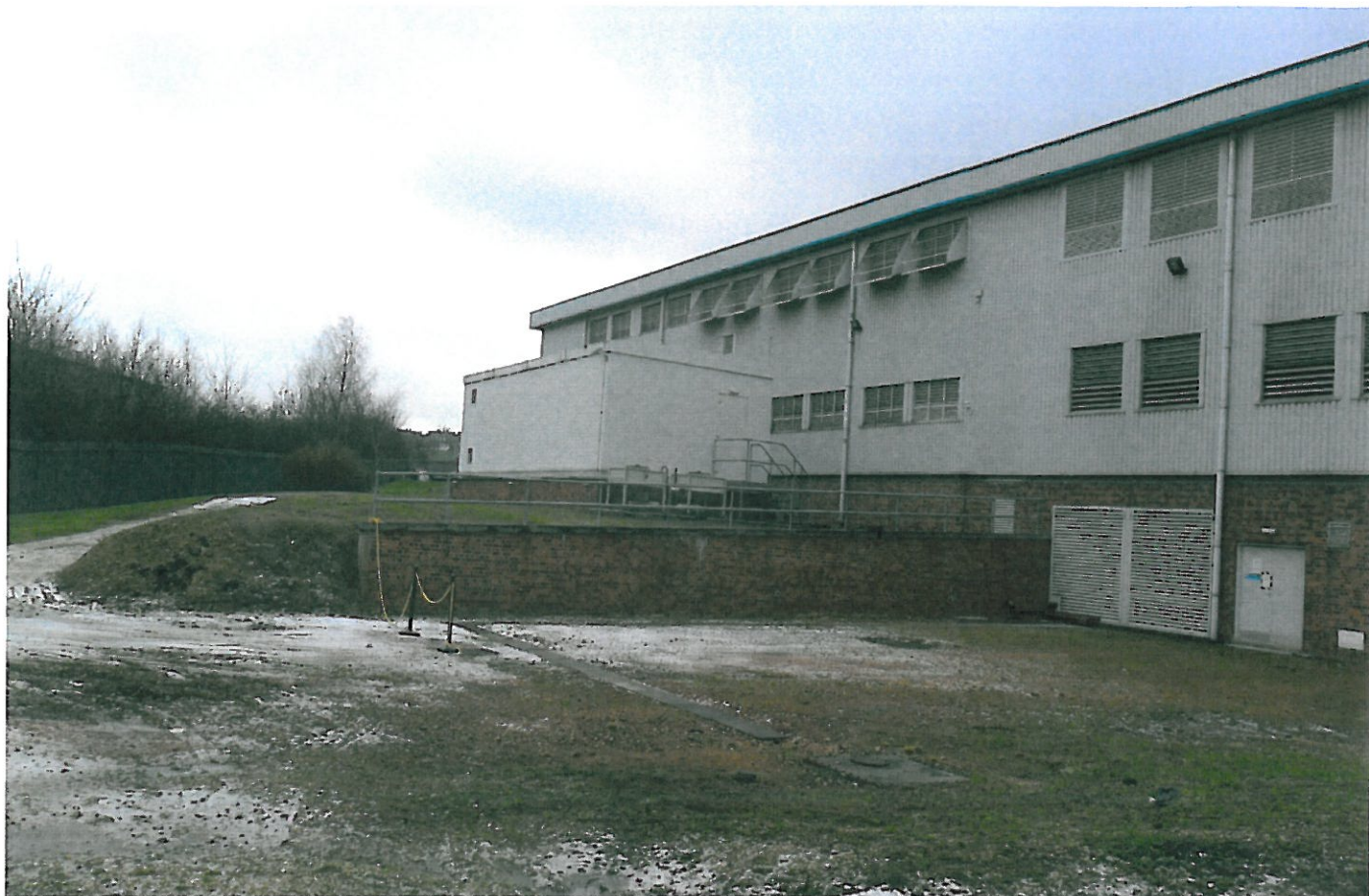
Photograph No. 5 – (North East Elevation)
