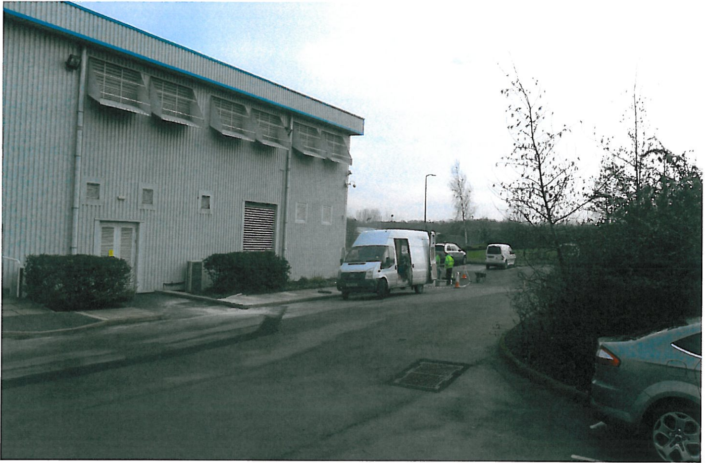
Photograph No. 9 – (South West Elevation)
