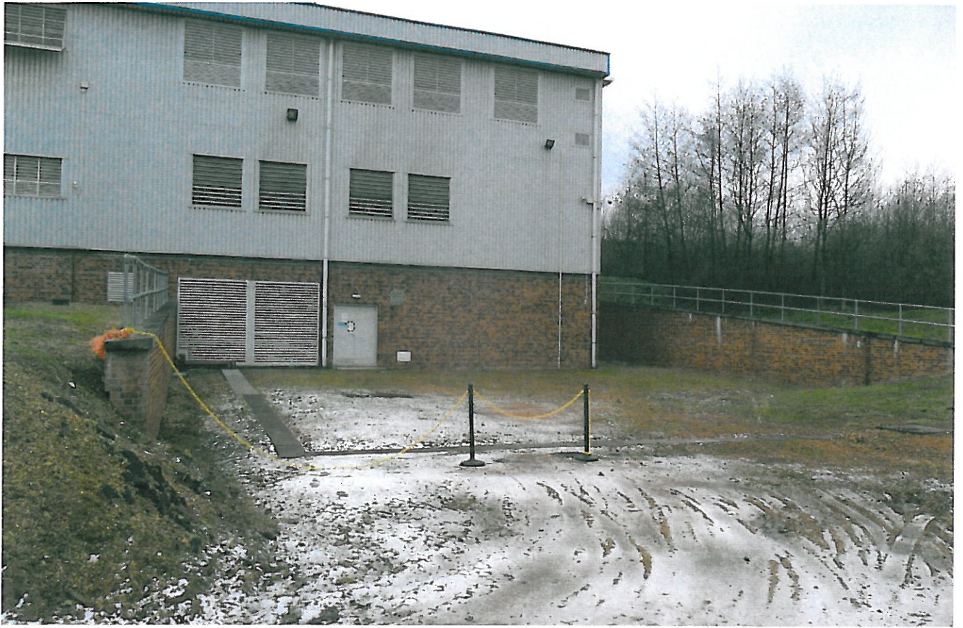
Photograph No. 1 – (North East Elevation)
