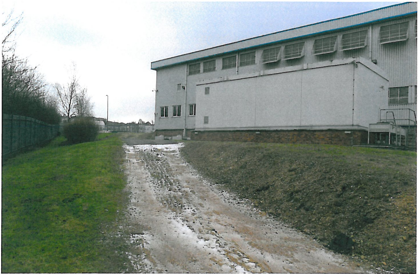
Photograph No. 3 – (North East Elevation)
