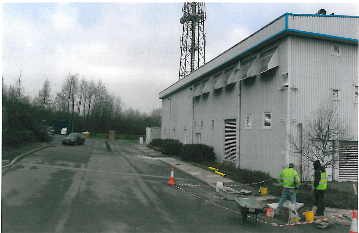
Photograph No. 8 – (South West Elevation)
