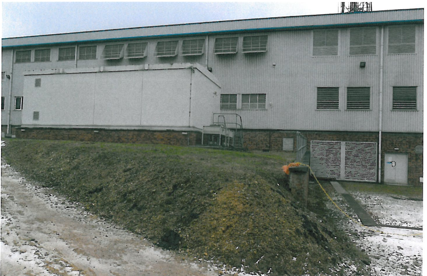
Photograph No. 4 – (North East Elevation)
