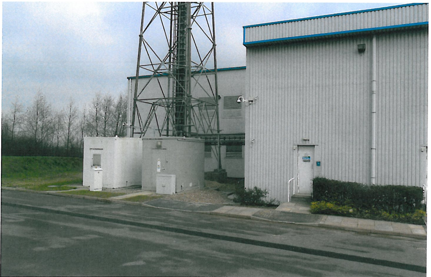
Photograph No.10 – (South West Elevation)
