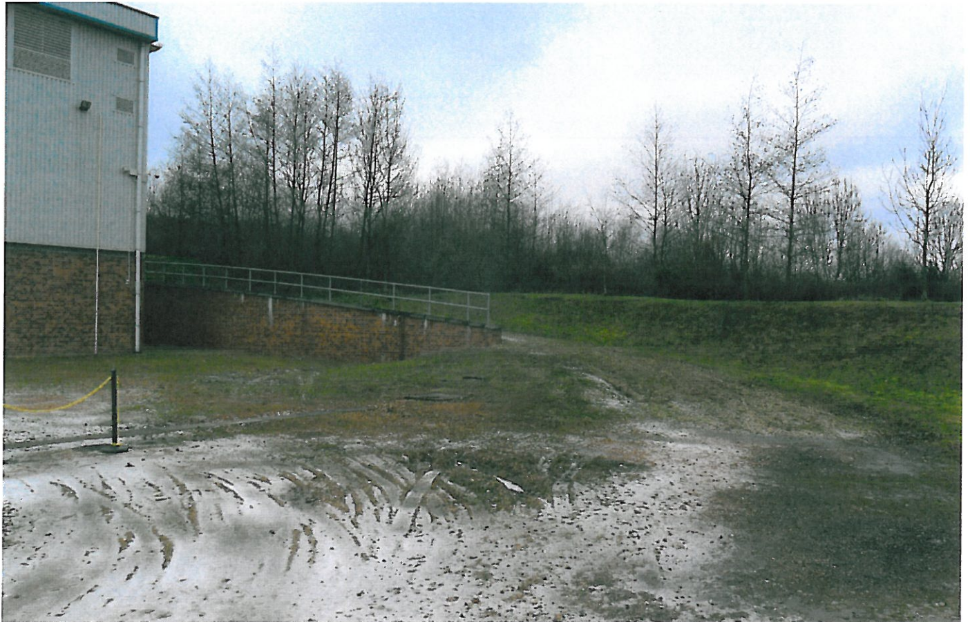
Photograph No. 2 – (North East Elevation)
