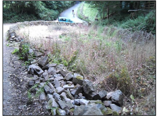
Photograph 2: The site viewed from the west
