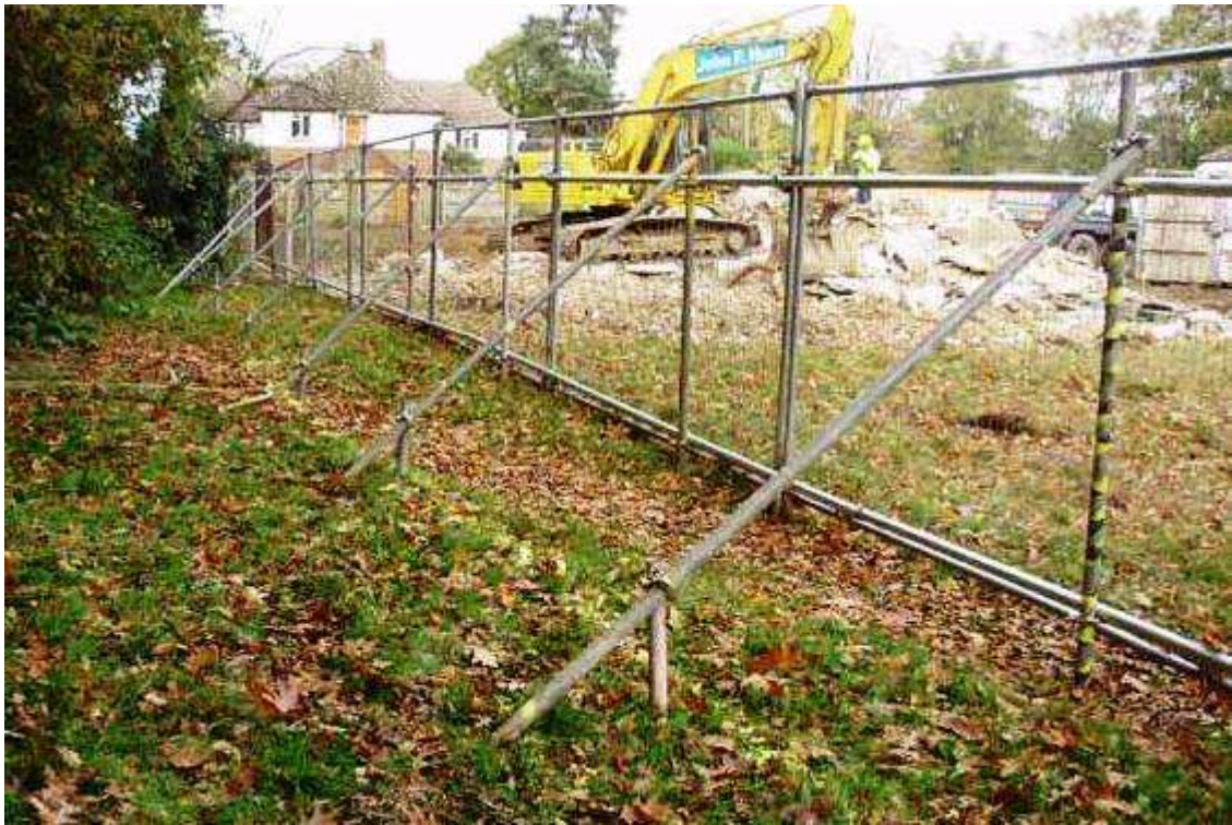
Figure 2: 'Photo of Fencing to BS 5837: 2012'.
