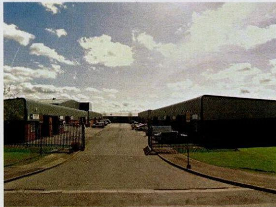
Goldthorpe Industrial Estate
