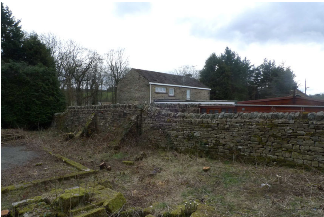
10 View of dry stone wall on Western boundary
