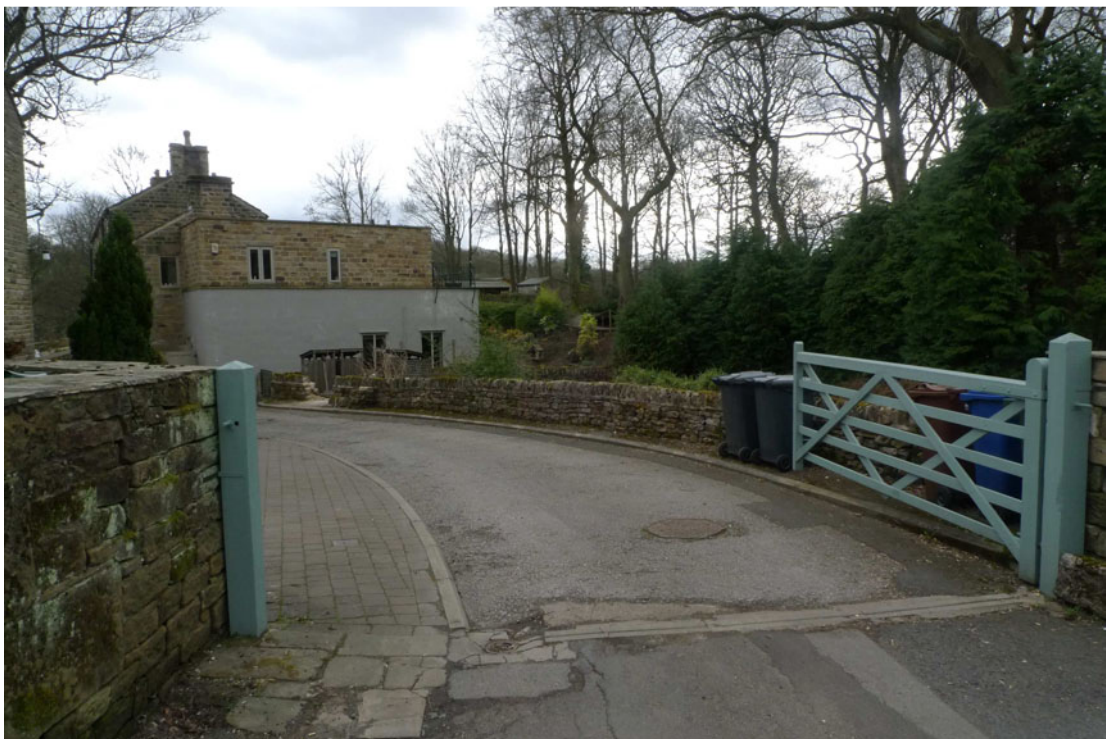
4 View looking SW to the Old Mill
